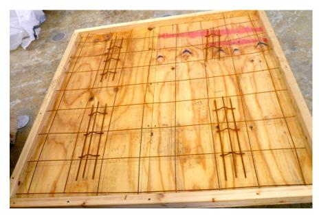
Figure 4.1: Impact Panel Formwork
