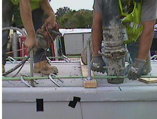
Figure 8. Photograph showing vibrator and concrete placement for bridge B0410 HCB.
