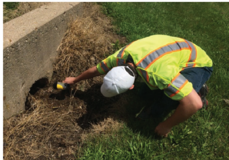
(e) Inspecting inside culvert with flashlight
