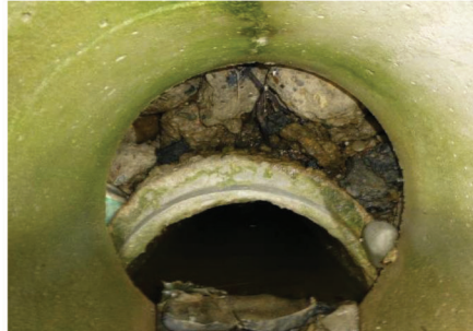
(b) End section detached allowing sediment and rocks to fall through
