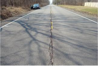
Figure 13. Cracking parallel to centerline joint of 26th Street, April 2014.
