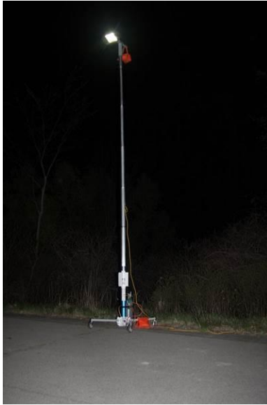
Figure 2-31. Floodlight with internal glare shielding with 70 W MH source.
