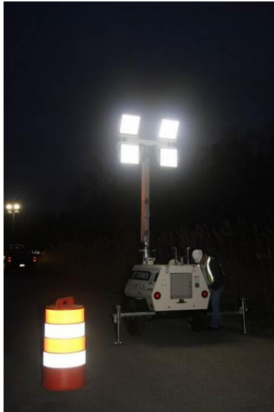
Figure 2-18. Light tower with four 270 W LED lights.
