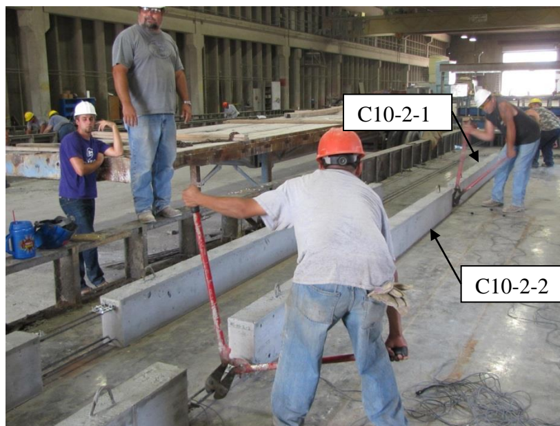
Figure 5.14 – Release of C10-2 Beams
