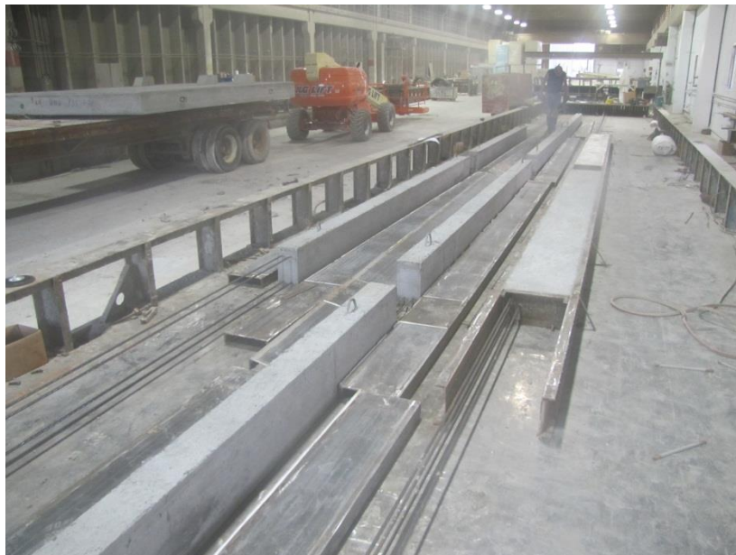
Figure 4.9 – Beams After Form Removal and Before Instrumentation
