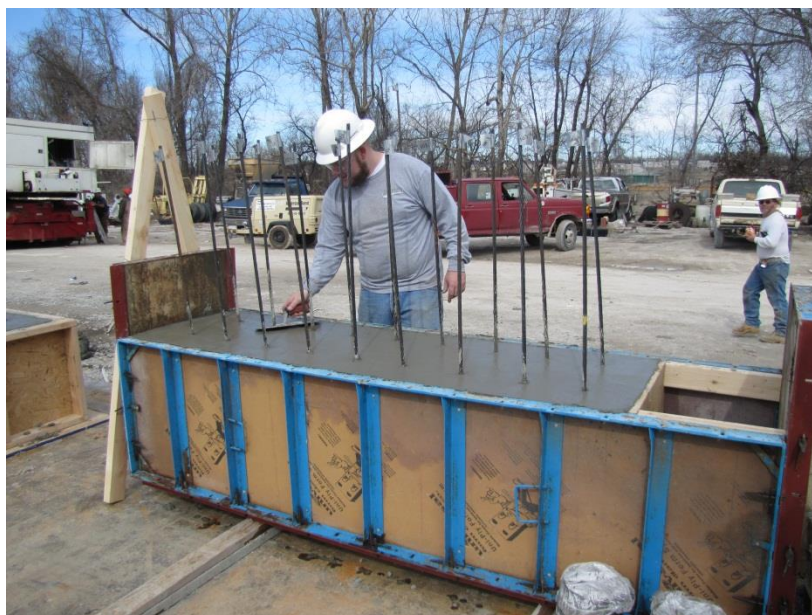
Figure 3.24 – Finished LBPT Specimen
