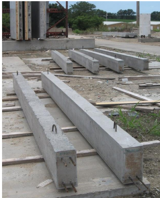
Figure 4.14 – C6 and S6 Beams in Storage Yard at Coreslab
