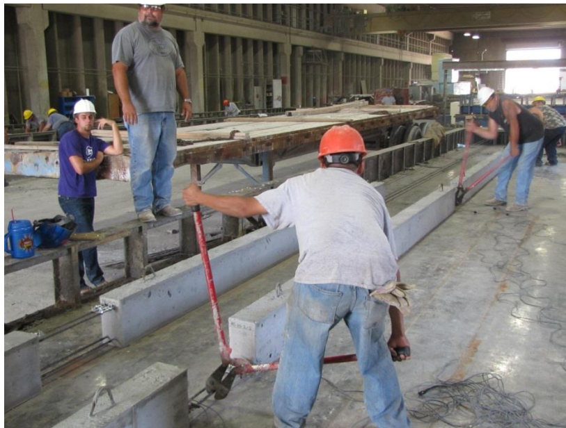
Figure 4.10 – Bolt Cutting Strands at Release
