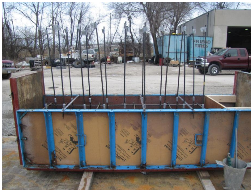
Figure 3.22 – LBPT Specimen Before Casting
