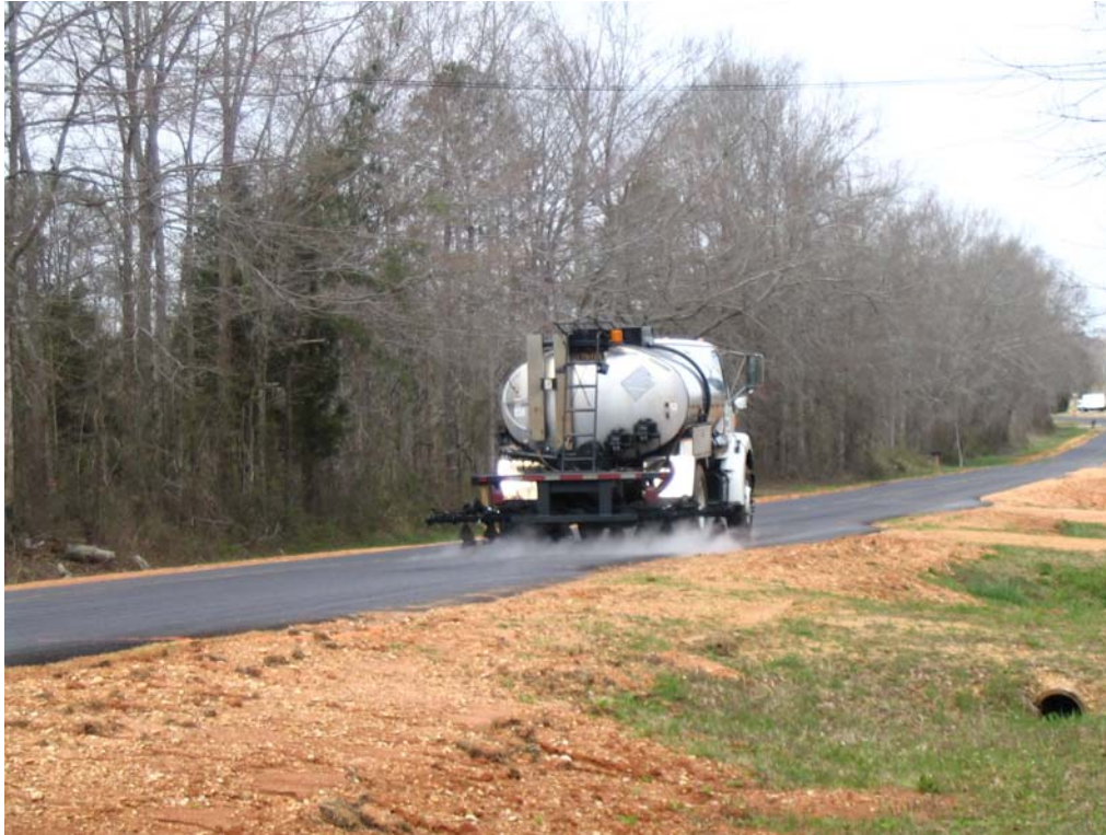
Figure 24. Application of CSS-1 Tack Coat on Project 5
