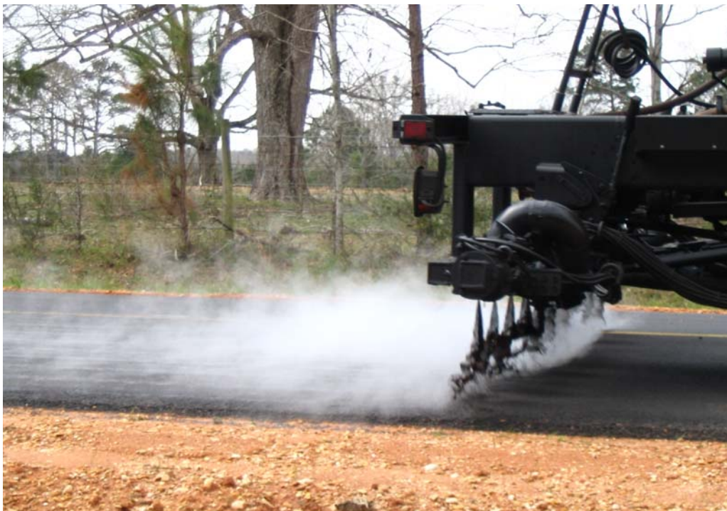
Figure 25. Close Up of Application of Tack coat on Project 5
