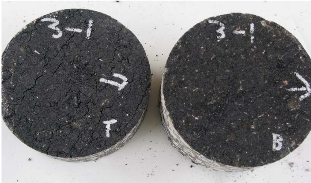
Figure 18. Core from Project 1 Showing Hairline Cracks in Surface Layer (left)
