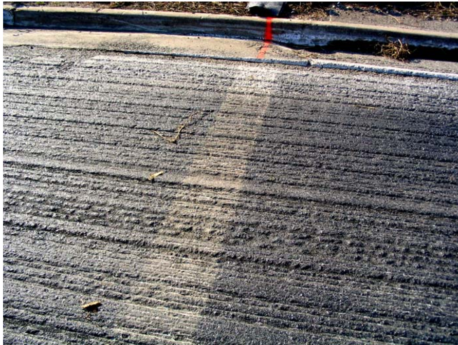
Figure 21. Photograph Showing Location Where Geotextile Pads Were Used to Measure Actual Tack Coat Application Rate
