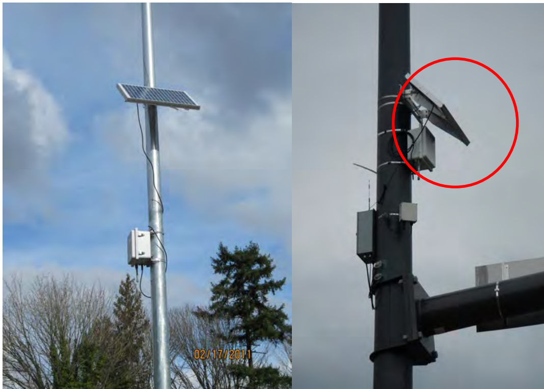
Figure 3-9. BlueTOAD sensor design and components
