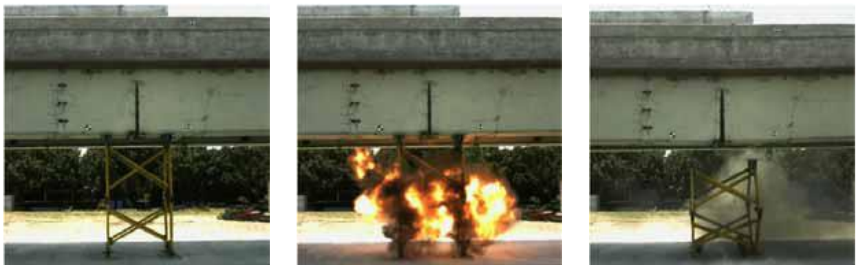
Figure 1-4. FSEL Second Bridge Fracture Test [Source: FHWA Report No.: FHWA/TX-10/9-5498-1]
