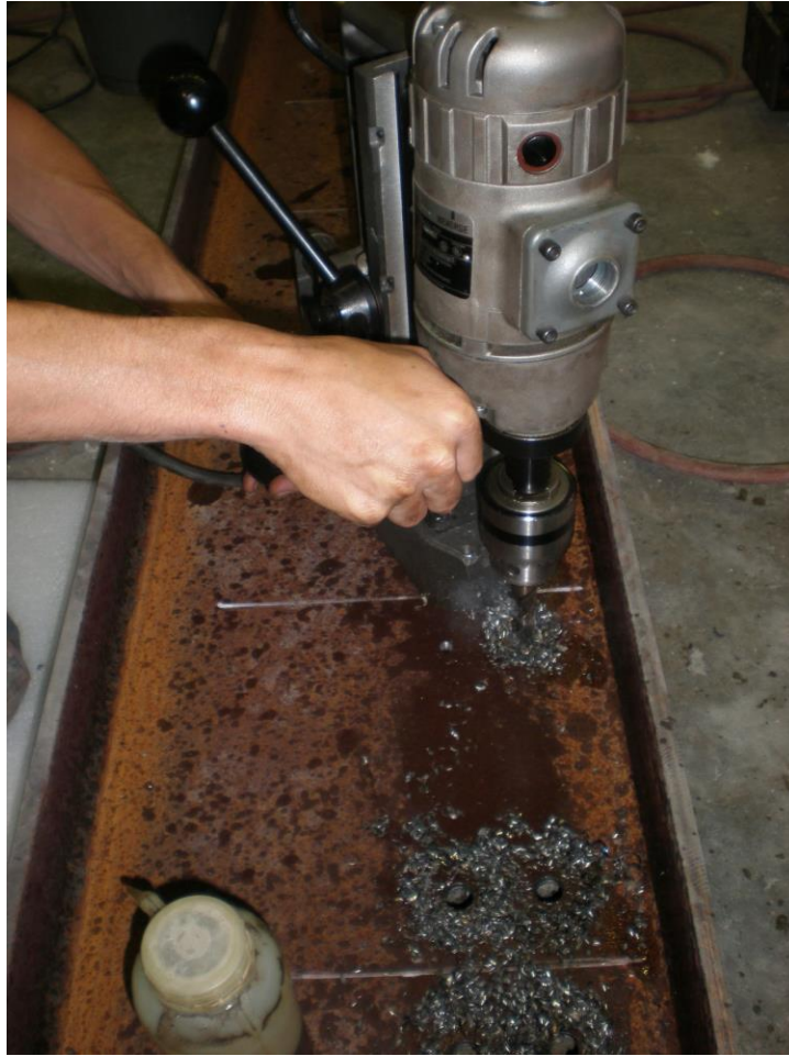
Figure 4-2. Drilling Girder Web for Connecting the Floor Beams
