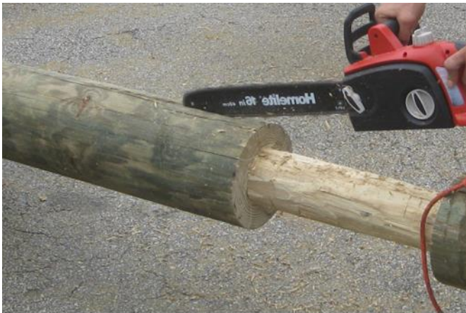
Figure 4.3: Preparing pile for GFRP sheet
