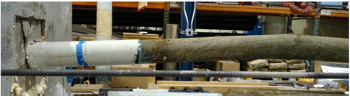
Figure 5.10: Failure of specimen 4 (2 inch deep damage filled with grout)
