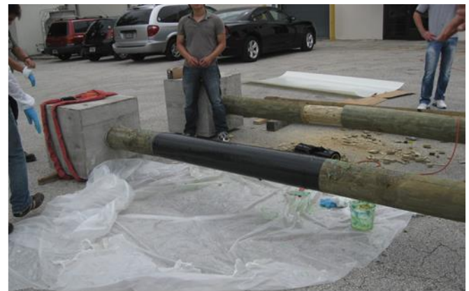
Figure 4.5: Holding GFRP sheet around the pile by Saran™ plastic wrap
