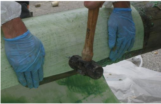
Figure 4.4: Wrapping GFRP sheet around the pile
