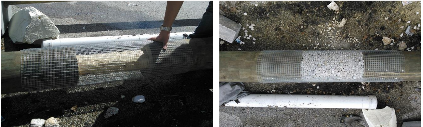
Figure 4.6: Wire mesh for holding aggregate in damage region
