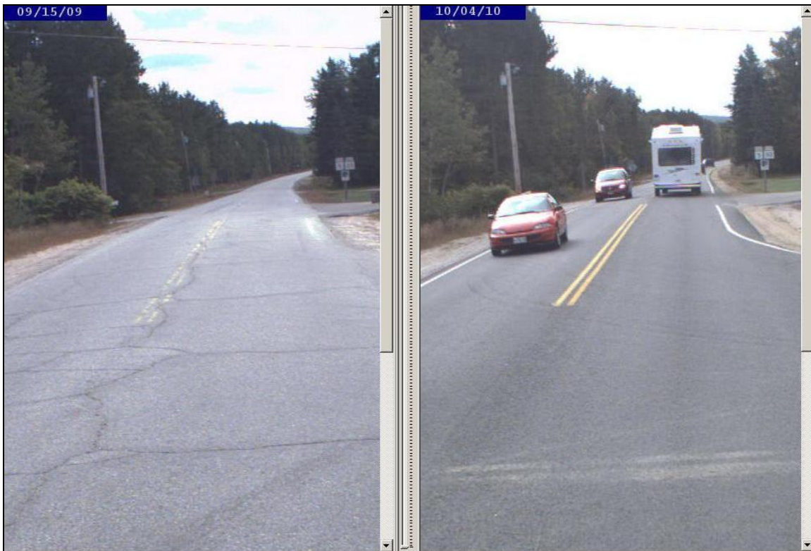
Construction Report 11-02 NovaChip Pilot Project –Route 5, Waterboro, Brownfield, & Fryeburg
