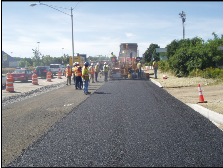
Figure 7 - Construction of 3" Open Graded Friction Course surface
