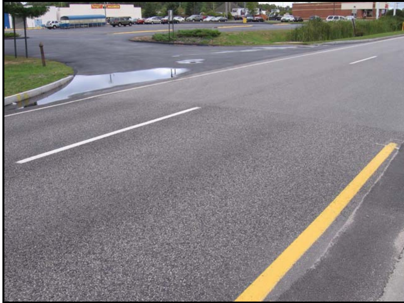
Figure 12 - Note difference between OGFC and Conventional HMA Surface
