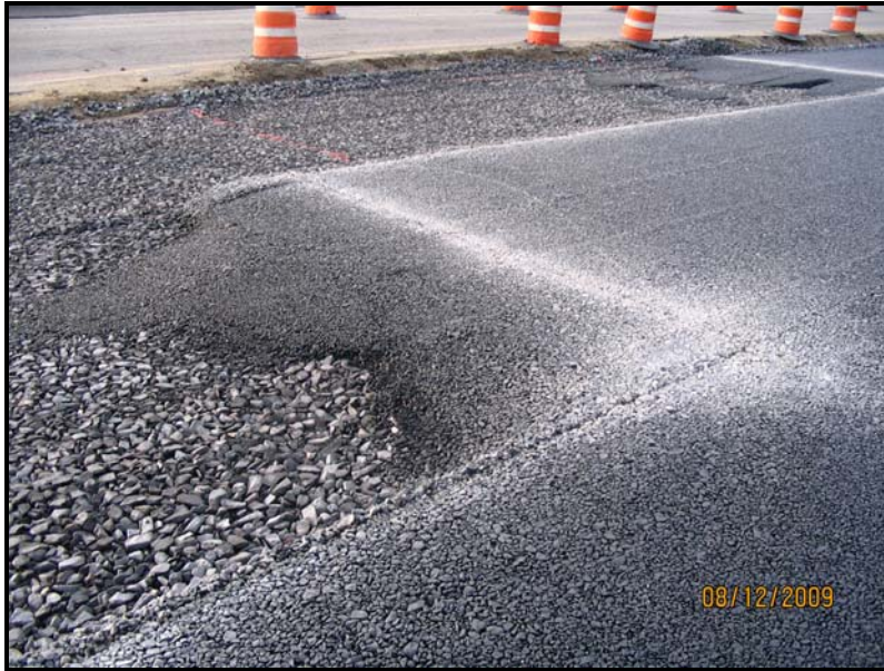
Figure 5 - Saw cutting of ATPB
