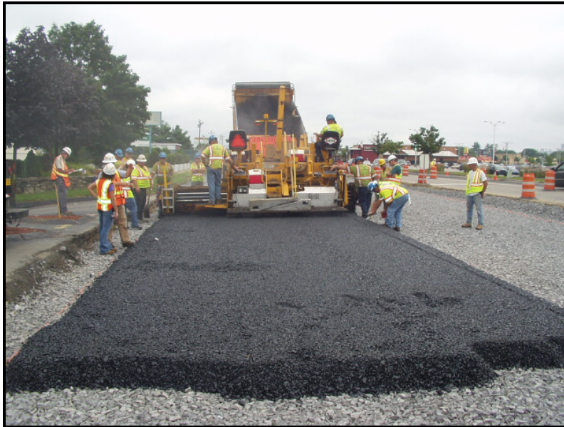
Figure 4 - Six inch Asphalt Treated Permeable Base placed on reservoir stone.
