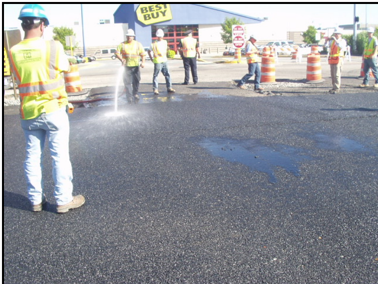
Figure 8 - Demonstration of ability to pass water.
