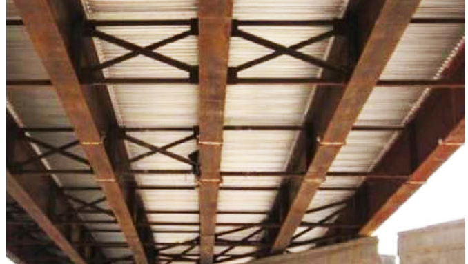
Cross-bracing system installed on a skew bridge.
