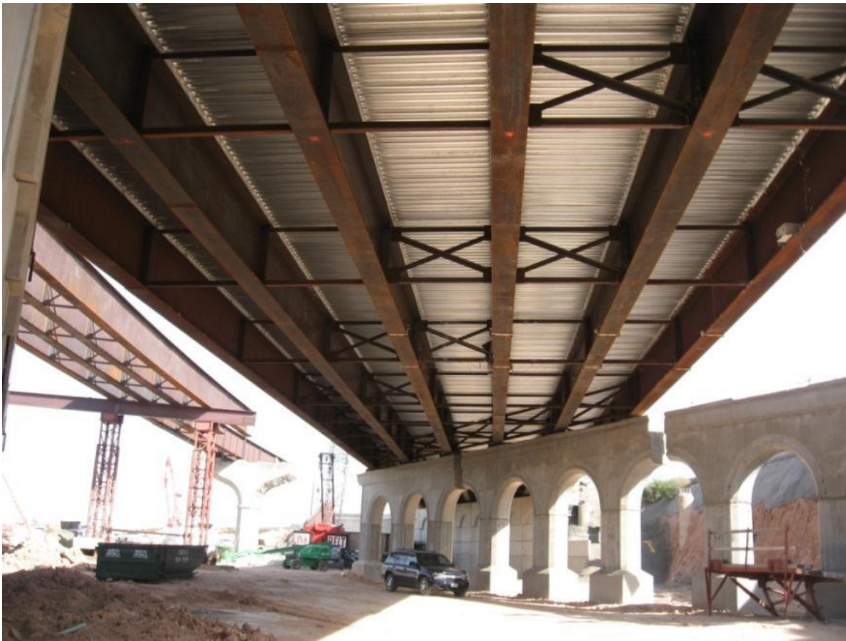
Figure 4.11: Lean-on bracing system in 19 th Street Bridge
