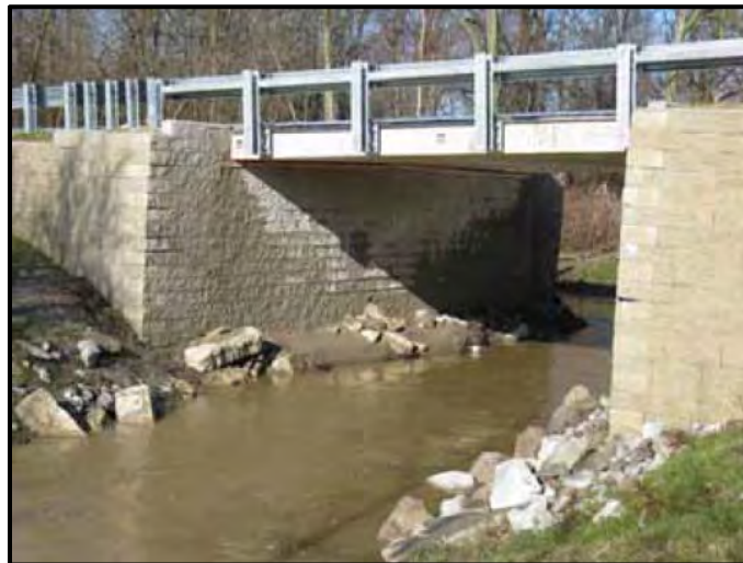
FIGURE 2.29 GRS Bridge System in Service
