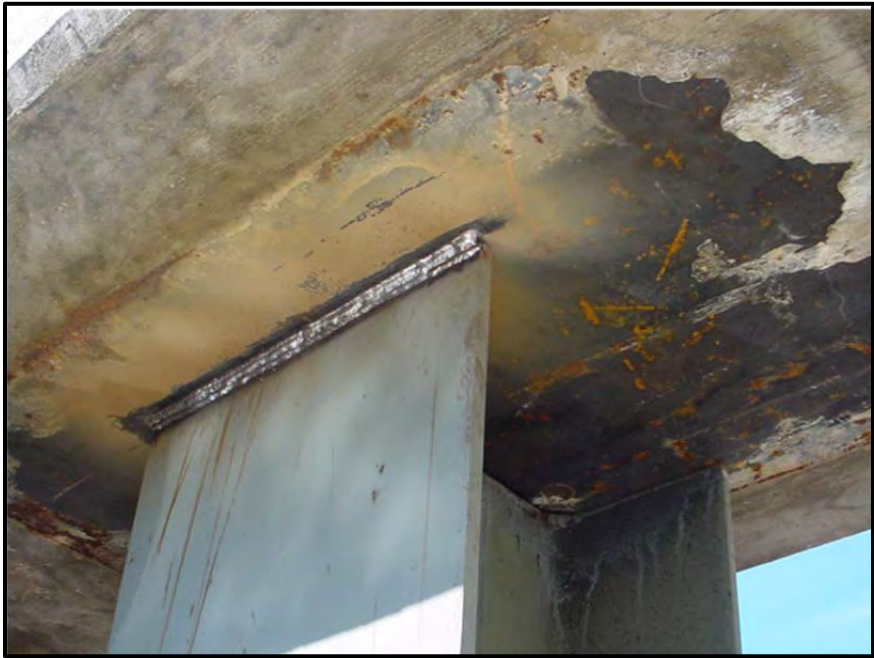
FIGURE 2.26 Welded Embedded-Plate Connection for Substructure
