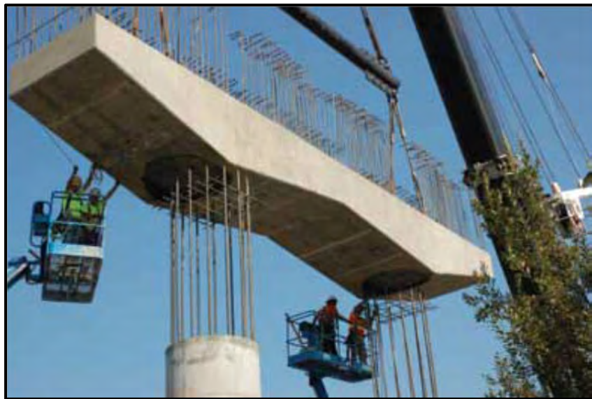
FIGURE 2.28 Placement of Precast Substructural Elements
