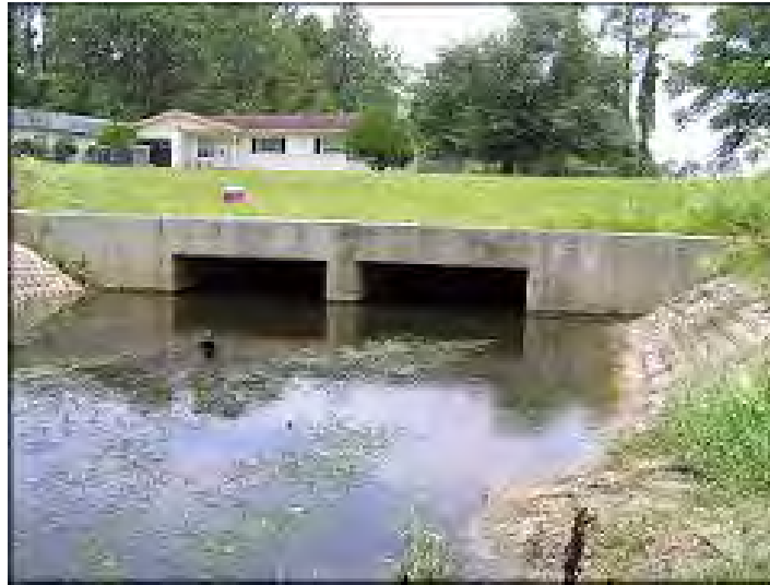
FIGURE 1.4 Box Culvert with Narrow Waterway Opening
