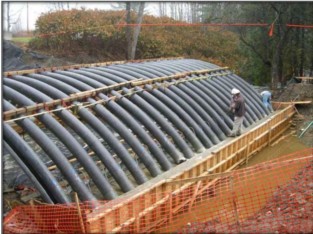
FIGURE 2.18 Bridge-in-a-Backpack Under Construction
