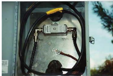
Feedline Lightning Arrester – Red Bluff
