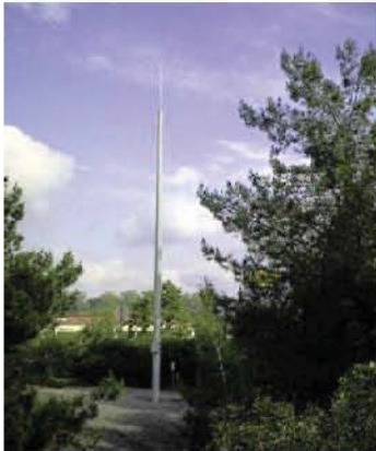
Antenna Installation – Red Bluff
