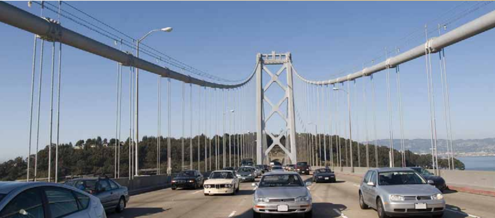
Bay Bridge in San Francisco, California
