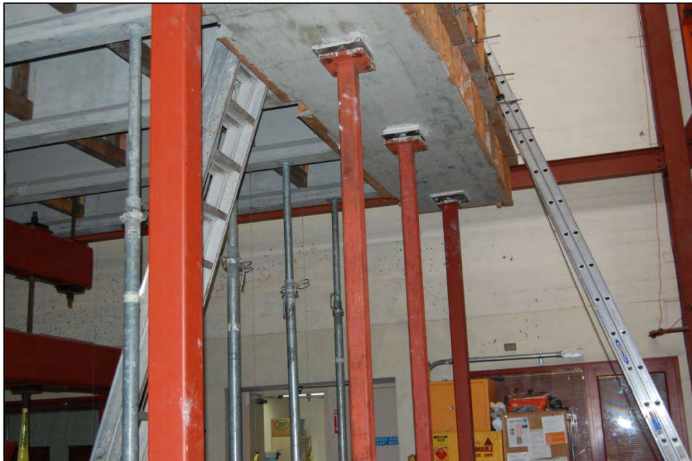
Figure 5.7: Temporary Support System Used Under Each Abutment
