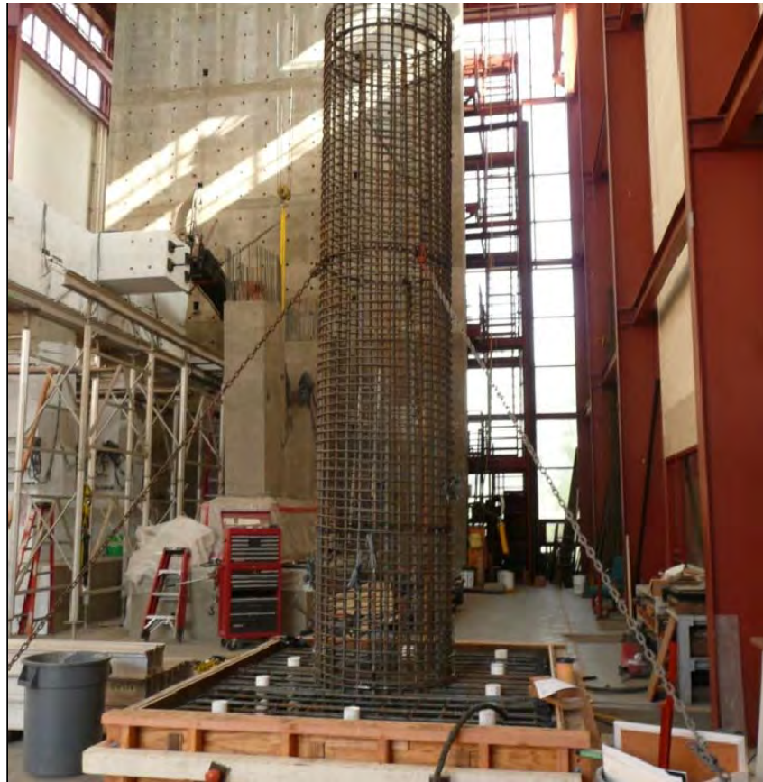
Figure 5.2: Completed Column and Footing Cage
