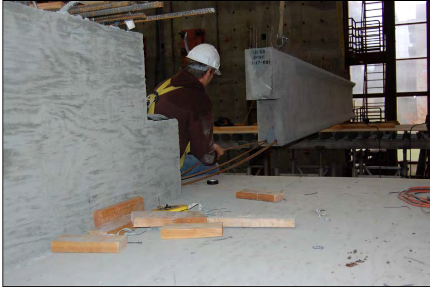
Figure 5.11: Pushing the Strands through the Girder
