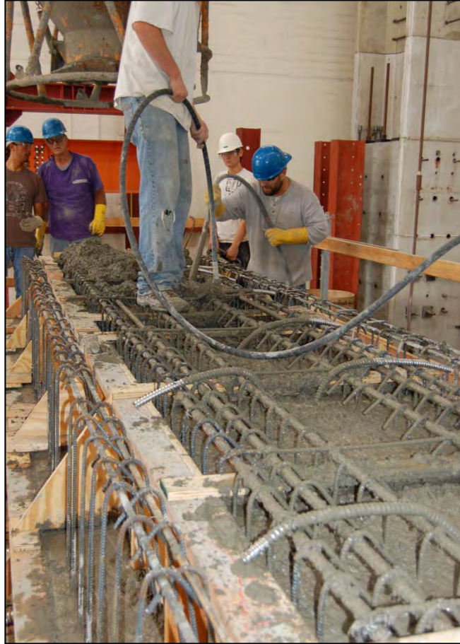
Figure 5.8: Casting of the Bent Cap
