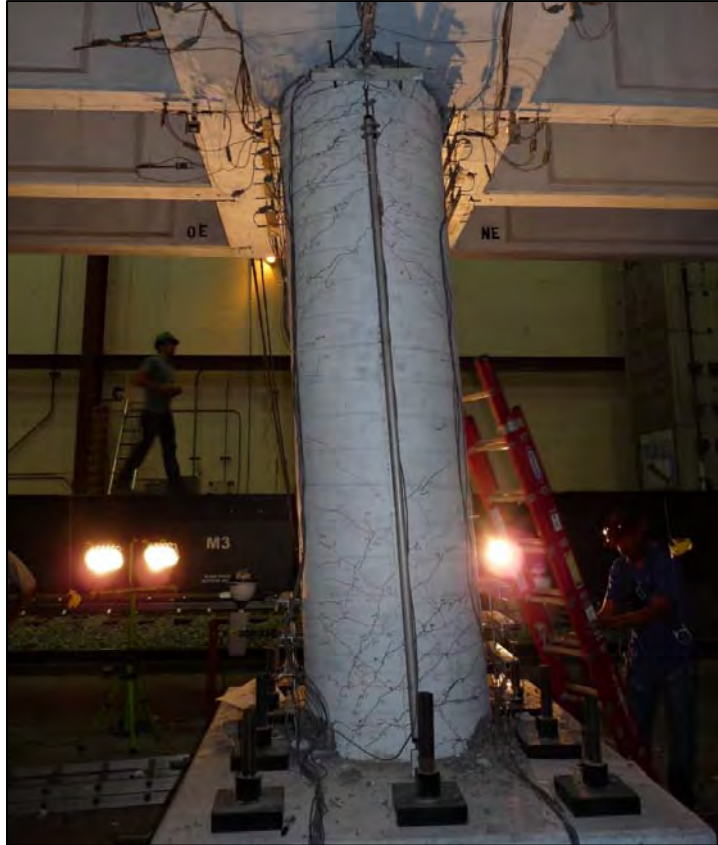
Figure 6.1: A Close-Up View of the Column Performance at +7.0 in. of Lateral Displacement ( \mu_{\Delta}=+10 )
