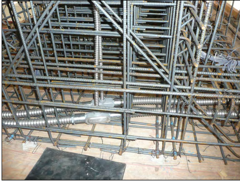
Figure 5.9: Routing of Bent Cap Ducts
