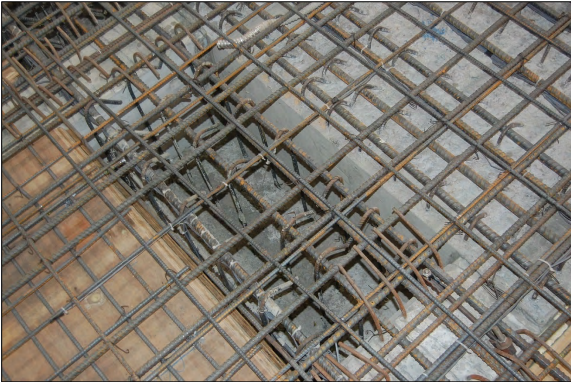
Figure 5.12: Partial Diaphragm Pour between Girders
