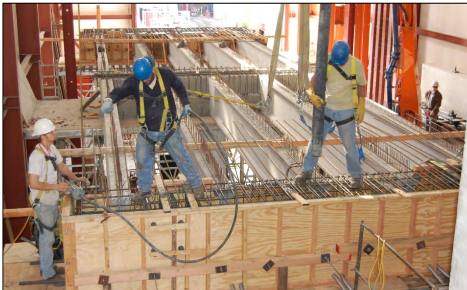
Figure 5.6: Casting of the North Abutment
