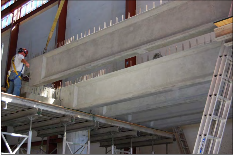
Figure 5.5: Installation of Southern Girders
