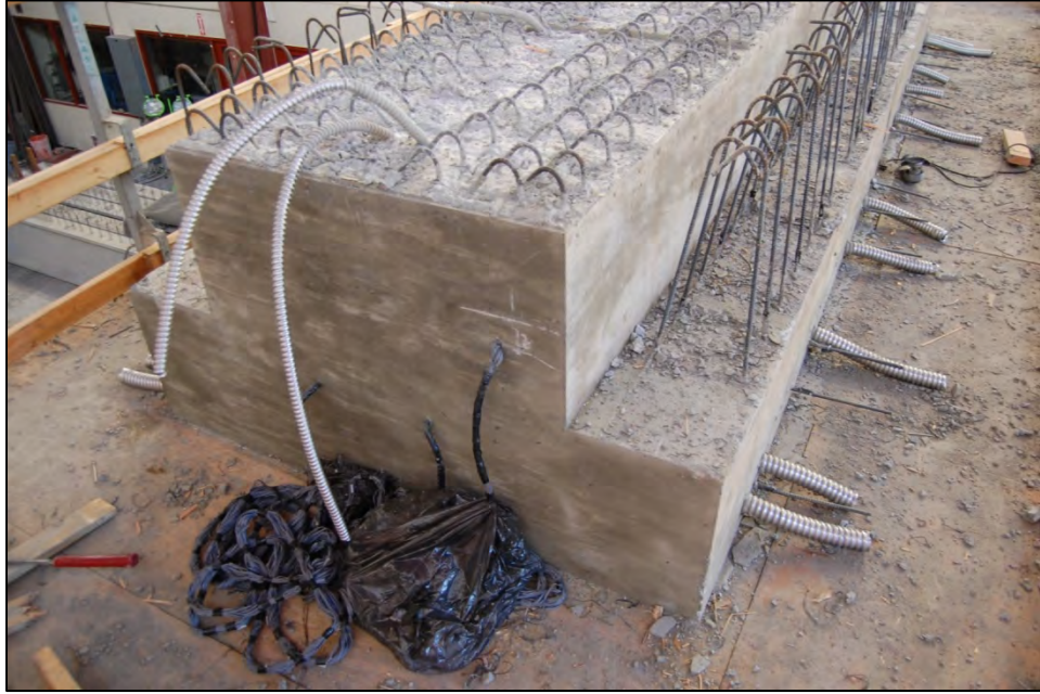
Figure 5.4: Completed Bent Cap Construction on Top of Column
