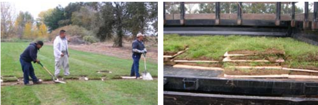
Figure 5.20 Lifting the cut sod onto boards using a shovel (left photo) and stacking the boards for transport on a trailer bed (right photo).
