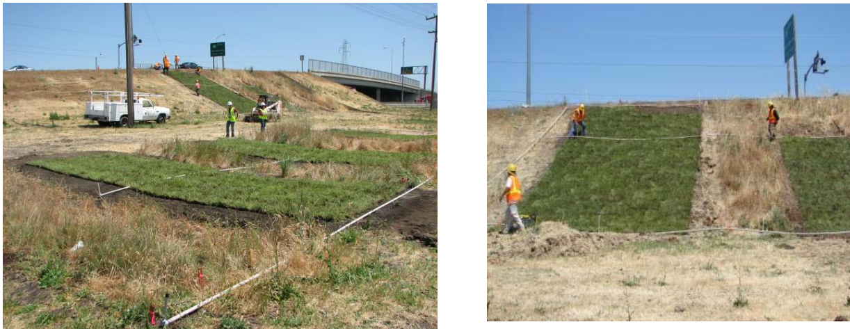
Figure 5.26 Irrigation line installation following transplanting the MSU Native Grass Sod–Delta on the drainage swale (left photo) and steep slope (right photo) areas on May 7, 2008.
