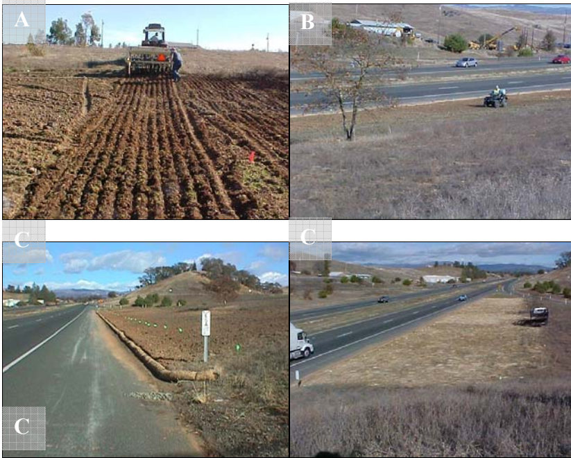
Figure 14. SR29 was drill seeded with native perennial grasses (A), sprayed with glyphosate to control weeds before native grasses emerged (B) and covered with straw to control excessive soil loss across the site and along the road edge (C) (November 2003).
