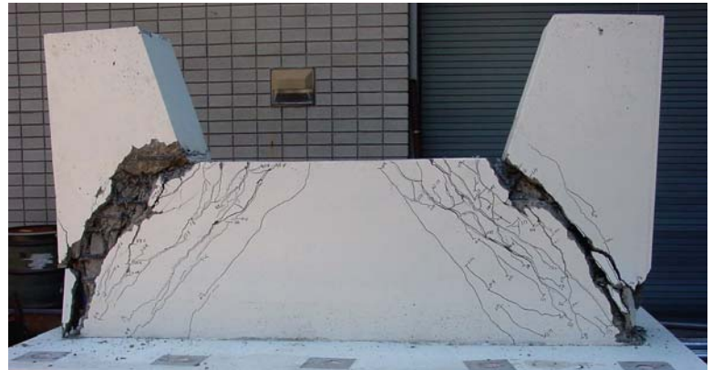
Figure 8-7. Expected damage to current external abutment sacrificial shear keys.
