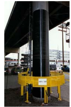
Figure 9-18. Carbon fiber jacking of bridge columns.
