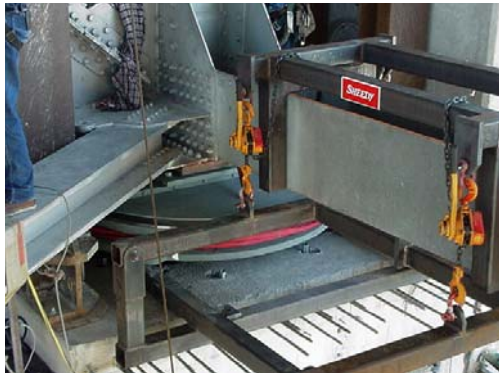
Figure 9-16. Installation of friction pendulum bearing on the Benicia-Martinez Bridge.
