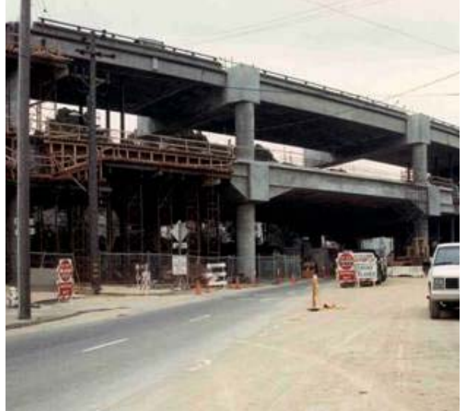
Figure 9-10. San Francisco double-deck viaduct retrofit.
