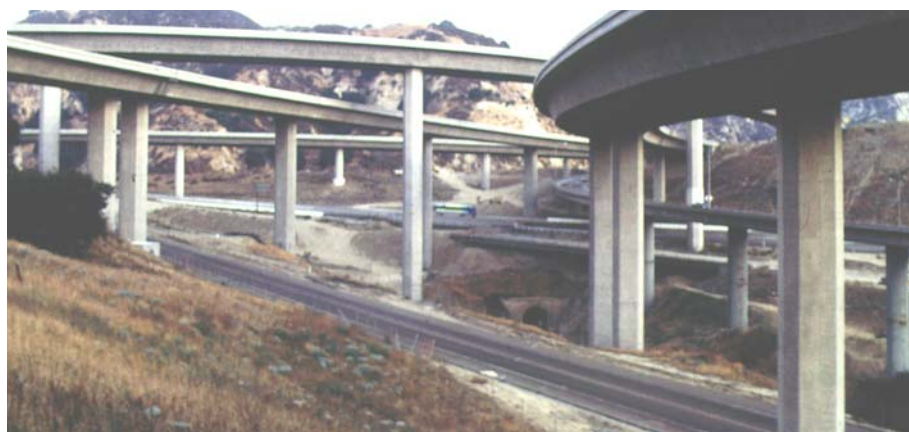
Figure 7-19. Reconstructed I-5 interchange.
