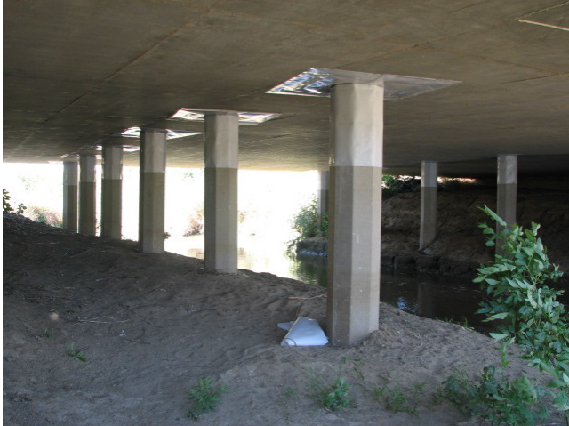
Figure 3. Highway structures with PTFE surface modification.
