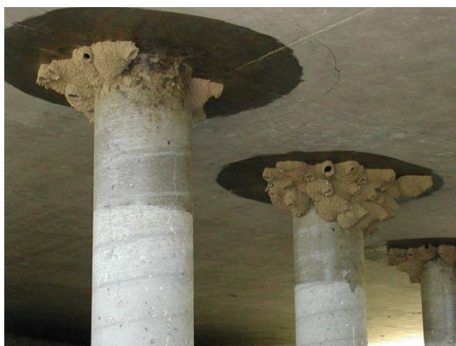
Figure 8. Completed nests on columns and overhead surfaces treated with silicone paint.
