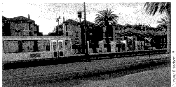
San Francisco Embarcadero light-rail station
