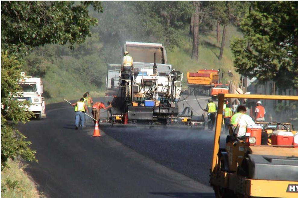
Figure 11-15 Roller Position During Application (Alvarez, 1992)
