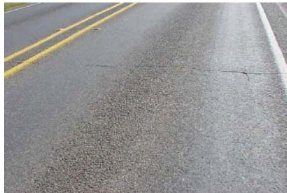
Figure 1-7 Transverse Cracks
