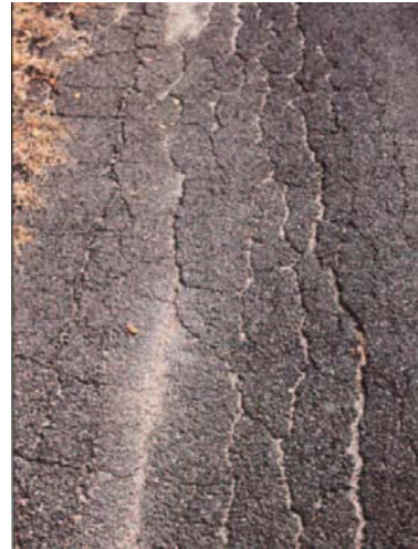
Figure 4-6 Edge Cracking
