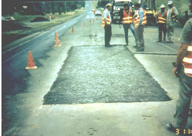
Figure 5-17 Dig Out Project
