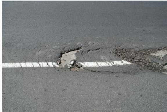
Figure 1-16 Delamination
