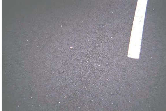
Figure 1-27 Segregation (seal coats)
