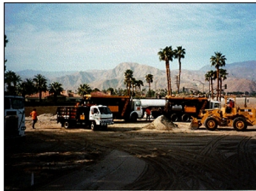
Figure 8-9 A Typical Stockpile and Project Staging Area
