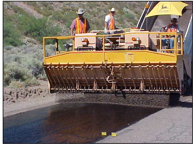
b) Spreading of Aggregate
