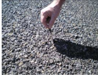
Figure 12-7 Polymer Modified Asphalt (PMA) Chip Seal
