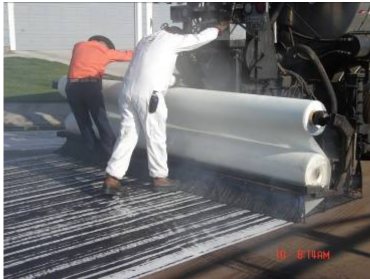
Figure 12-11 Truck Mount Application of Paving Mat
