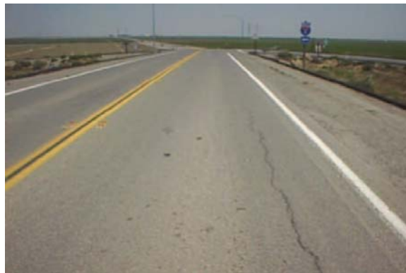
Figure 1-5 Longitudinal Cracks
