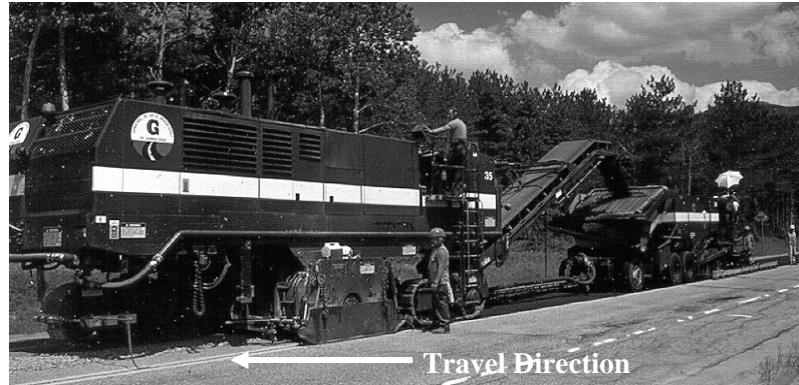
Figure 13-6 Two-Unit CIR Train in Operation (FHWA 2003)
