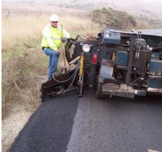
Figure 11-13 Paving the shoulder of Rt. 84 with BWC Type O using a shoulder backing machine in 2007.
