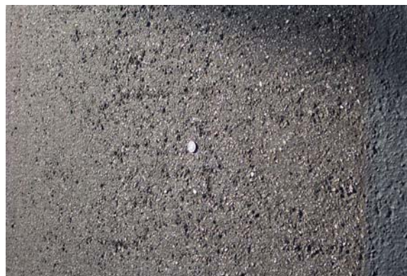
Figure 1-26 Rock loss
