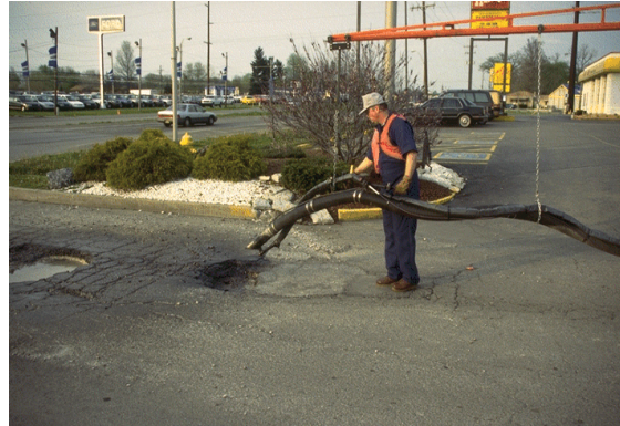
Figure 5-13 Application of Tack Coat
