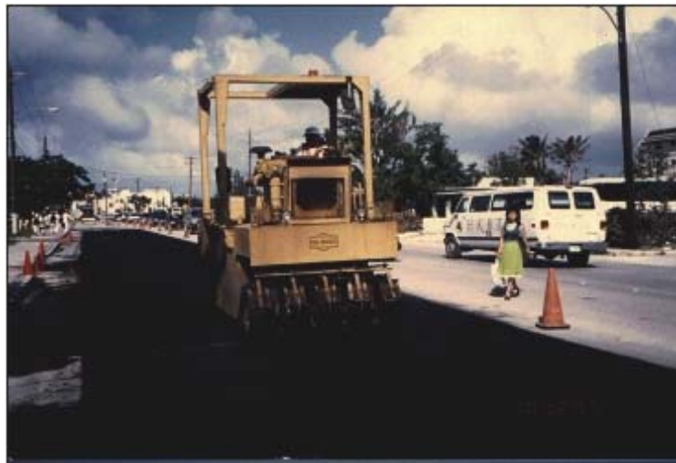
Figure 9-25 Rolling a Slurry Surfacing
