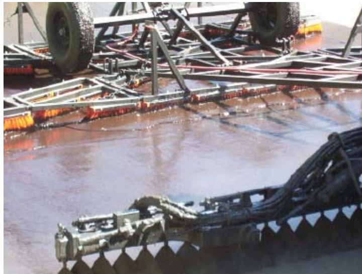
Figure 7-12 Scrub Seal Application
