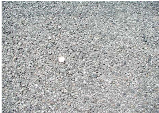
3 year old 3/8" OGAC. Suitable surface for fog seal and rejuvenator seal with application rates as high 0.12 gal/sq yd.
