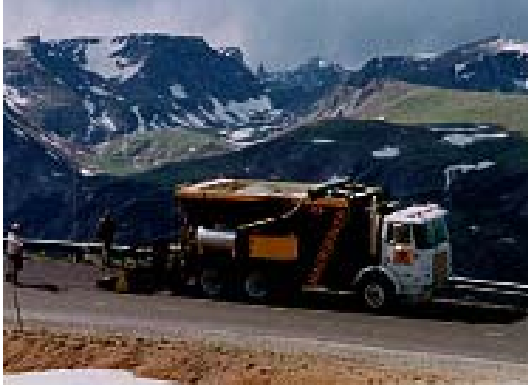
Figure 8-7 Slurry Surfacing Machine
