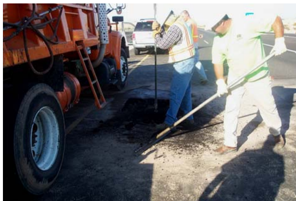
Figure 5-6 Throw and Roll Patching
