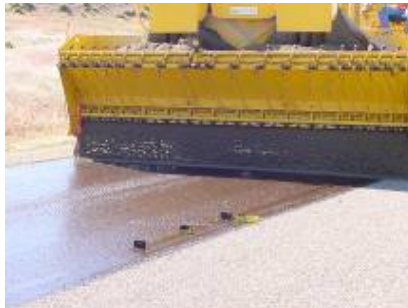
Figure 12-17, 18, 19 Scrub Seal Construction
