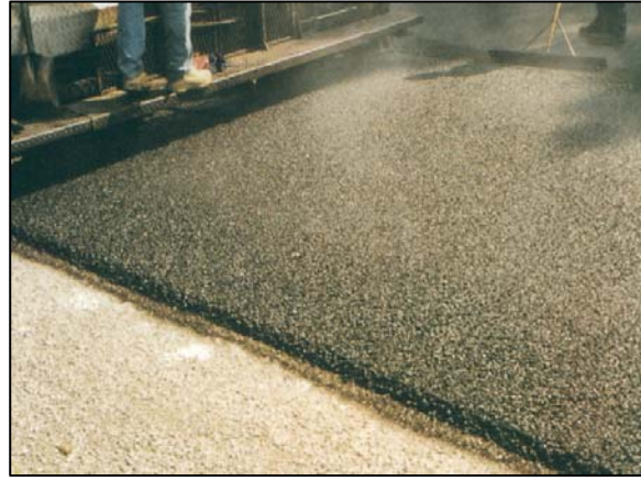
Figure 11-12 Freshly Laid BWC (Alvarez, 1992)
