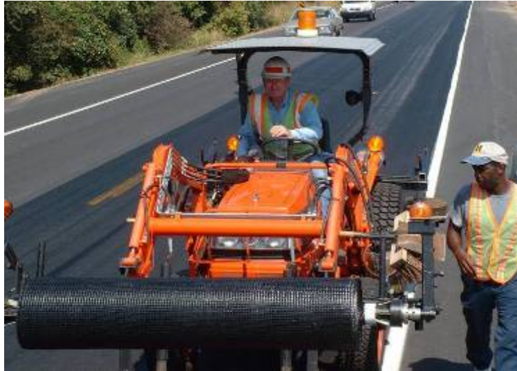
Figure 12-12 Tractor Mount Paving Grid Installation
