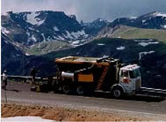
Figure 9-7 Slurry Surfacing Machine
