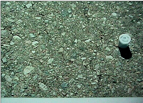
Dry, aged DGAC with open surface texture suitable for fog or rejuvenator seal with application rates typically ranging from 0.08-0.10 gal/sq yd at 50/50 dilution
