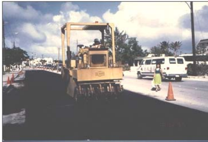
Figure 8-19 Rolling a Slurry Surfacing
