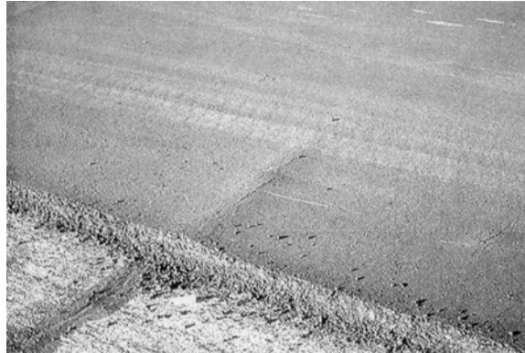
Figure 1-15 Overlay Bumps
