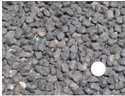
Figure 12-6 Asphalt Rubber Chip Seals
