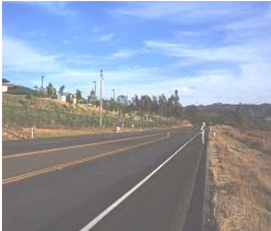
a) High Quality Longitudinal Joint
