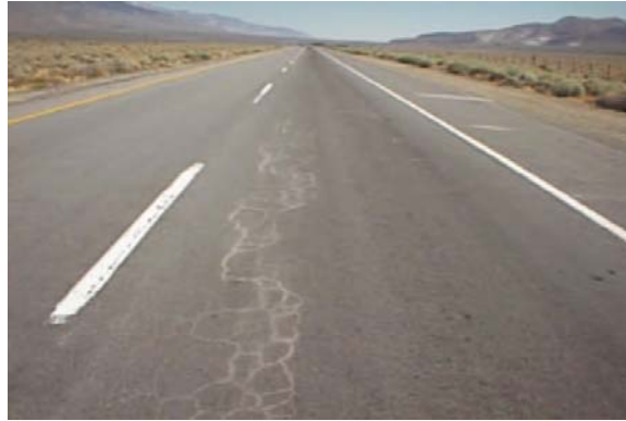
Figure 1-6 Fatigue Cracks
