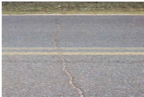
Figure 1-8 Reflective Cracks
