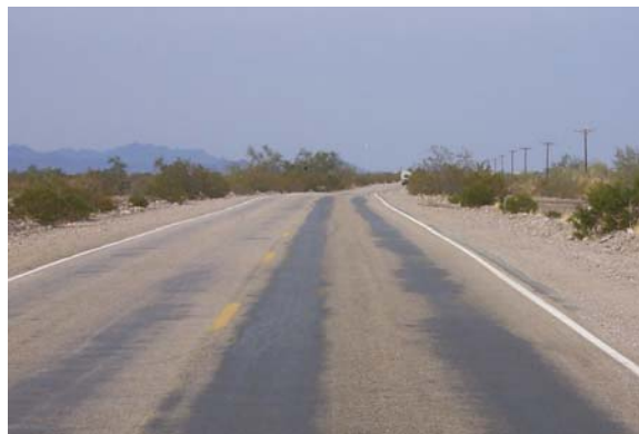
Figure 1-25 Bleeding (HMA)
