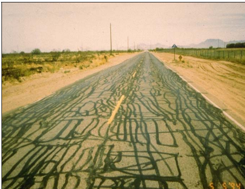
Figure 4-21 Excessive Sealant
