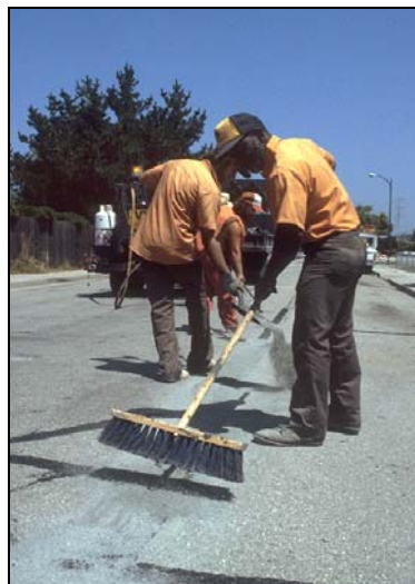
Figure 4-20 Brooming Blotter Coat Over a Treated Crack
