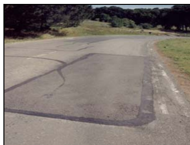
Figure 5-16 Edge Seal Application
