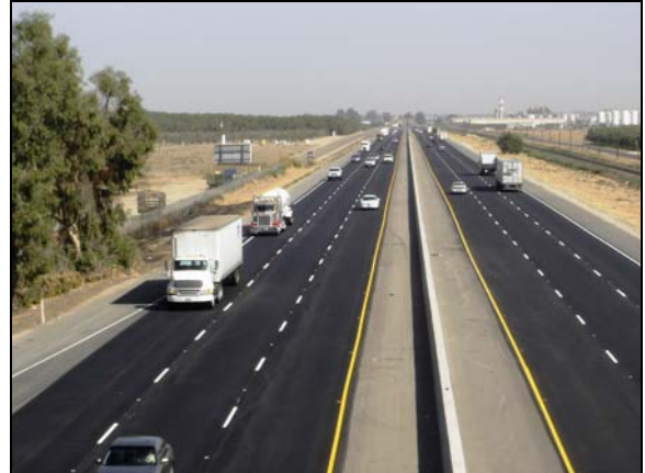
Figure 11-6 District 6 Rt. 99, The northbound lanes, or right-hand side, are BWC Gap Graded and the southbound lanes are RBWC Open Graded. Constructed in 2005
