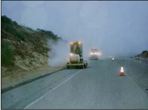
Figure 7-16 Brooming Process, Shown on a Shoulder Seal
