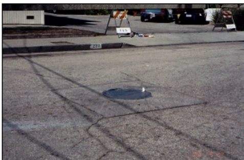
c) Cover Utilities with Kraft Paper
