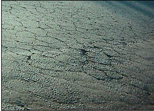
Figure 4-1 Fatigue Cracking
