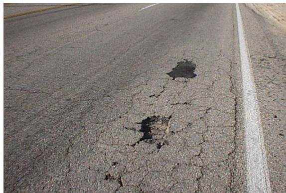
Figure 1-17 Potholes
