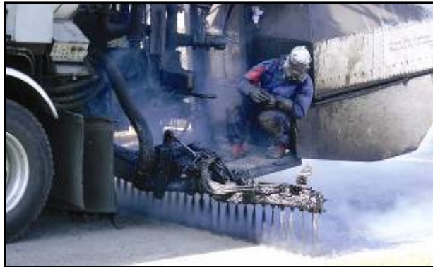
Figure 12-14 Asphalt Rubber Binder Being Applied
