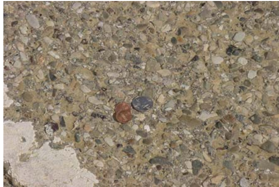
Figure 1-21 Polished Aggregate
