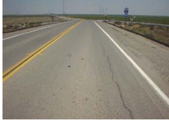
Figure 4-2 Longitudinal Cracking
