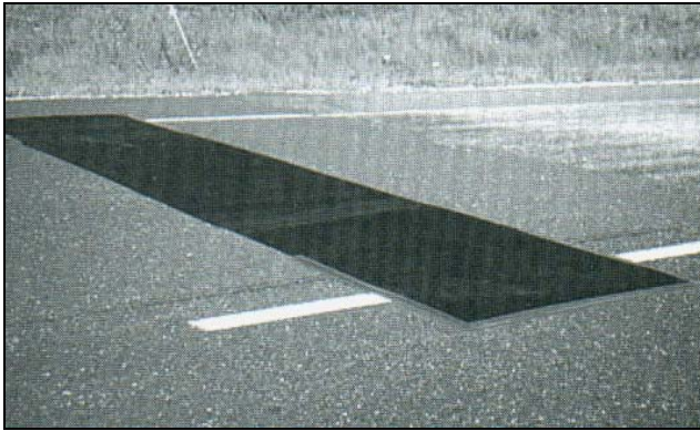
Figure 7-8 Start and Stop Passes on Roofing Felt (Transverse Joints)
