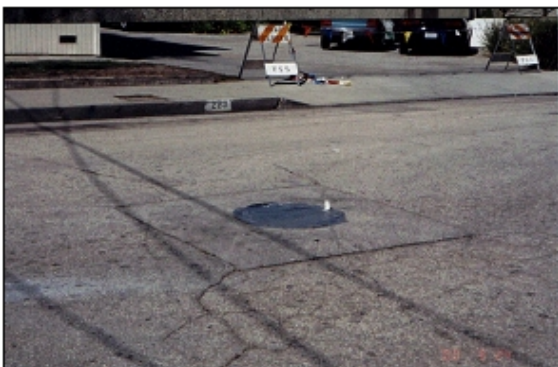
c) Cover Utilities with Kraft Paper
