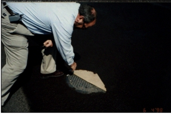
e) Peel Off Paper Covering Once Treatment has Cured
