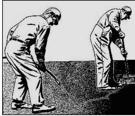
Figure 4-17 Manual Crack Cleaning
