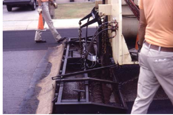
Figure 8-8 Slurry Seal Box with Augers
