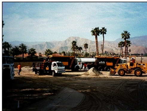
Figure 9-12 A Typical Stockpile and Project Staging Area
