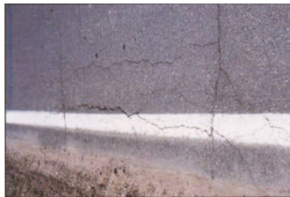
Figure 1-10 Edge Cracks
