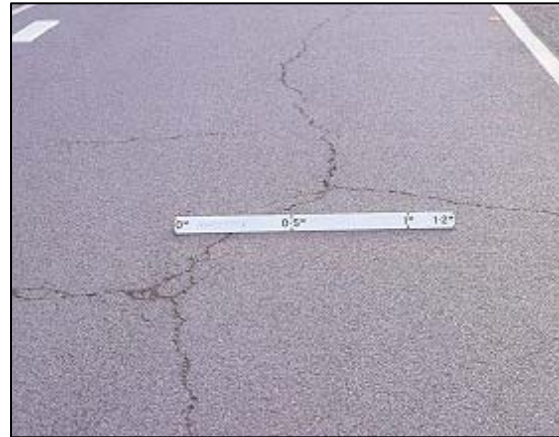
Figure 4-4 Block Cracking
