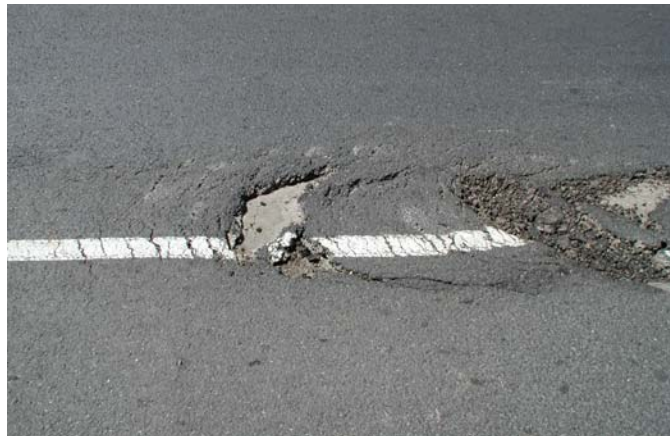
Figure 4-7 Slippage Cracking
