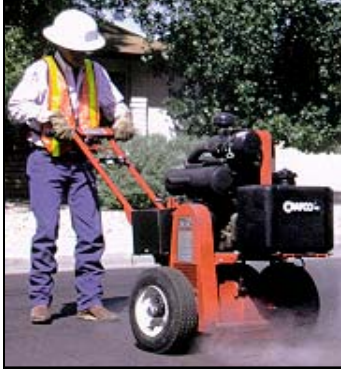
Figure 4-16 Crack Routing Operation
