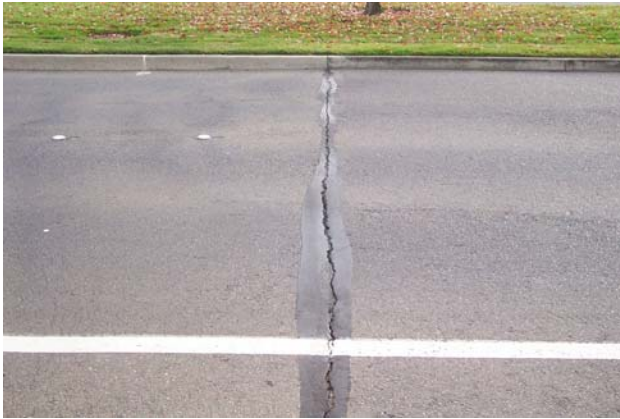
Figure 4-5 Reflection Cracking
