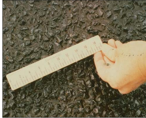
Good application of fog seal to new chip seal.
