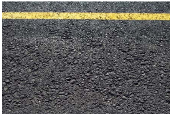
Figure 1-23 Segregation (HMA)
