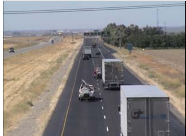
Figure 11-6 District 6 Rt. 99, The northbound lanes, or right-hand side, are BWC Gap Graded and the southbound lanes are RBWC Open Graded. Constructed in 2005
