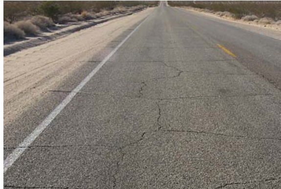
Figure 1-9 Block Cracks
