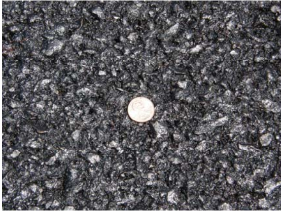
Good application of polymer modified rejuvenating emulsion at 0.10 gal/sq yd on gap graded rubber.
