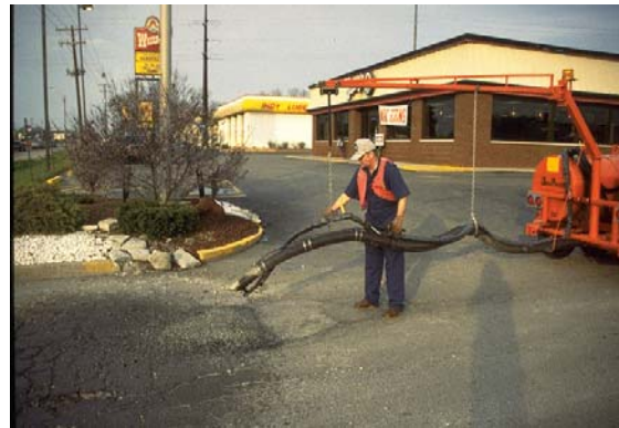
Figure 5-13 Application of Tack Coat
