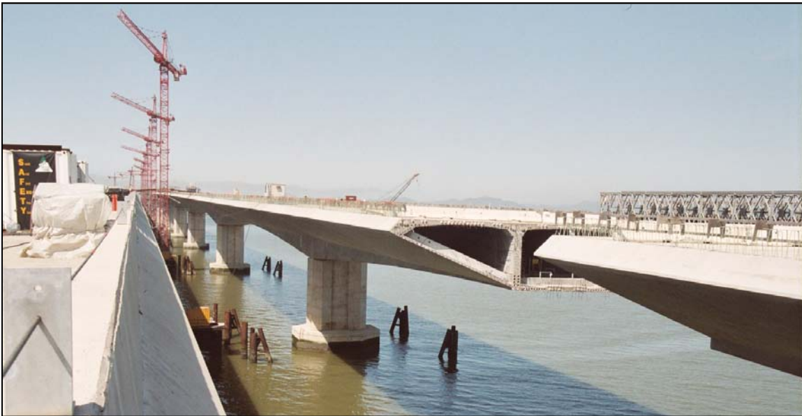
Figure 4-22 San Francisco Oakland Bay Bridge Skyway under Construction
