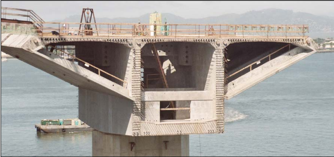
Figure 4-24 - San Francisco Oakland Bay Bridge Skyway Pier Section
