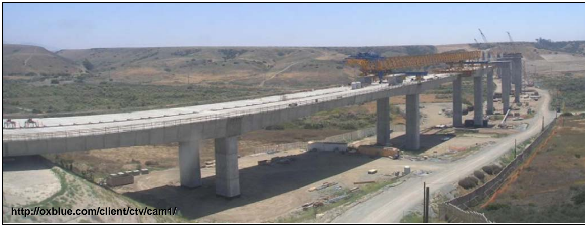
Figure 4-1 Otay River Bridge under Construction
