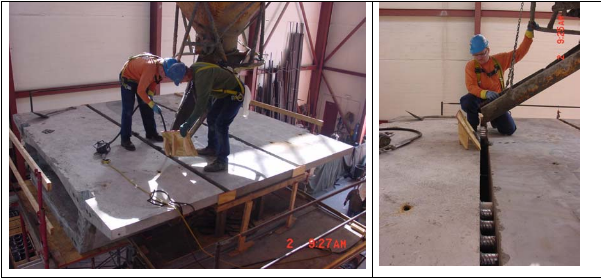
Figure 9.15 Pouring 3" closure gap
