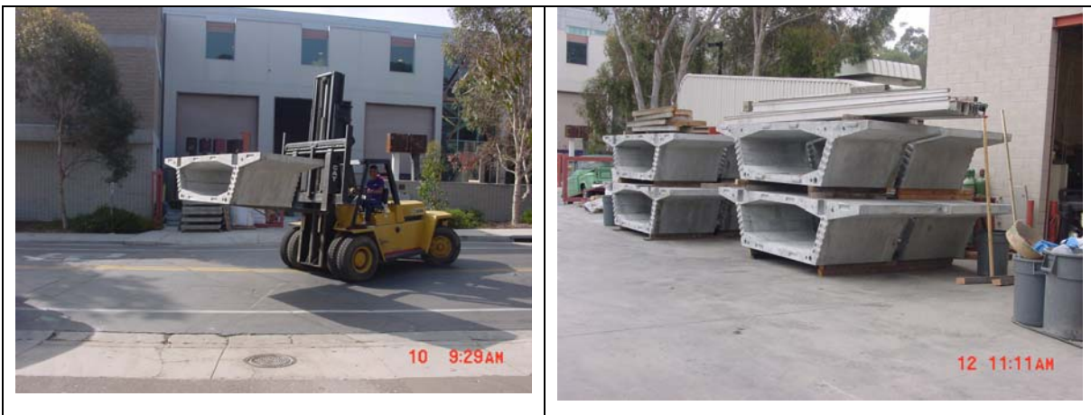
Figure 9.12 Unloading and storage of segments awaiting placement
