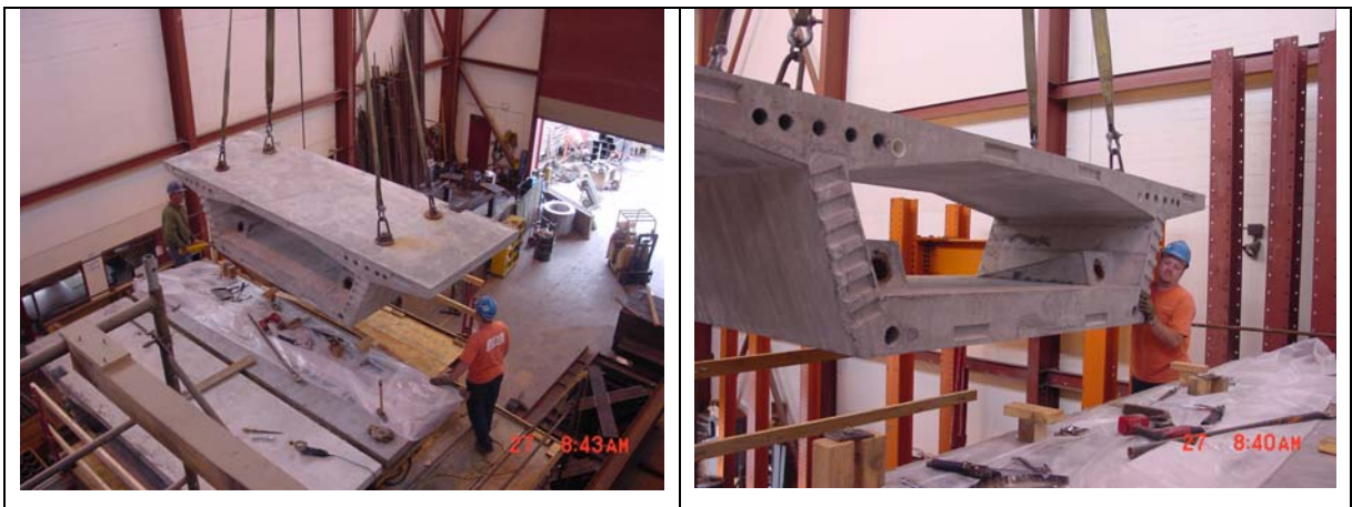
Figure 9.14 Continuing placement of 1 st pair of segments
