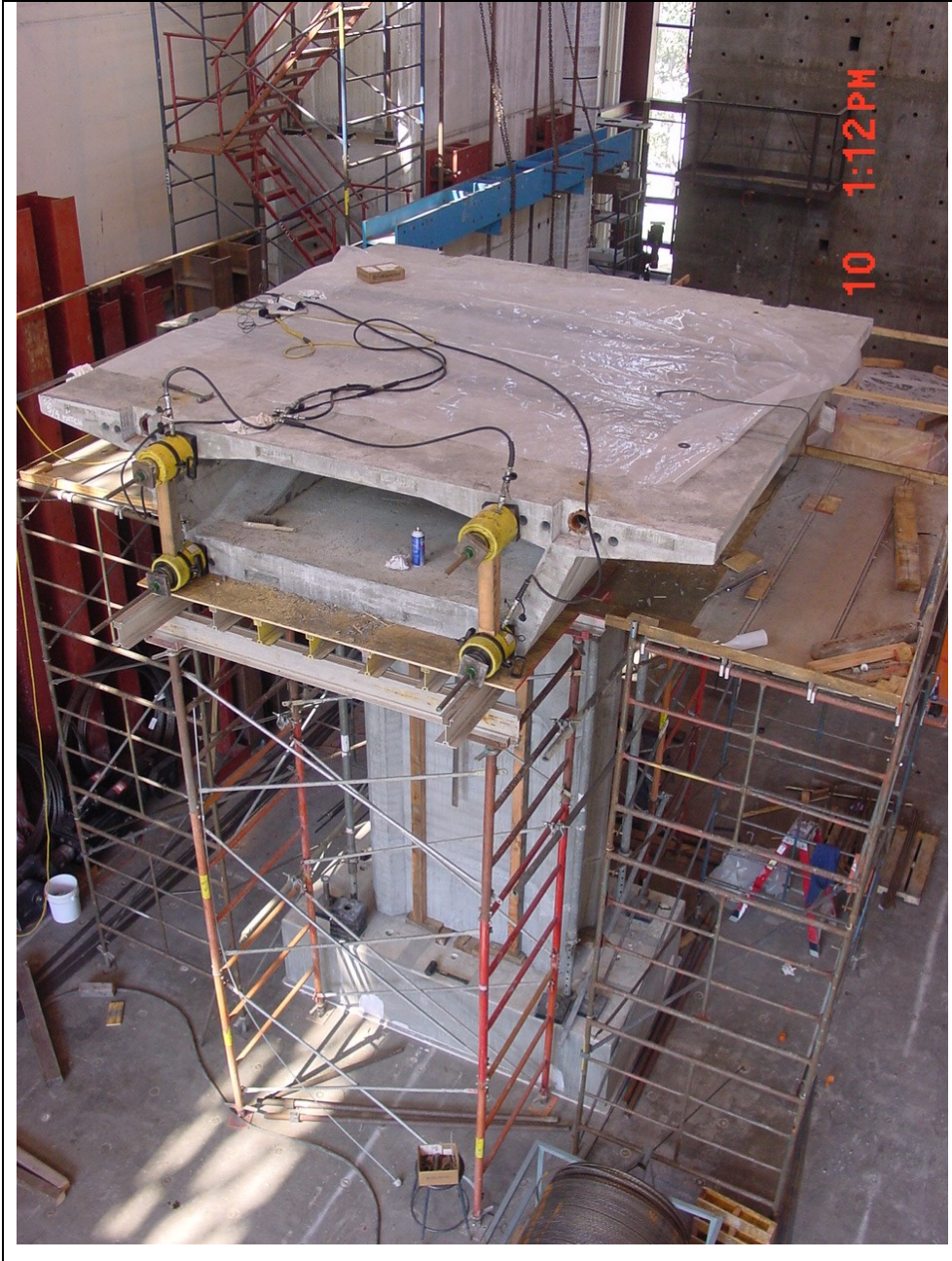
Figure 9.16 1 st pair of segments in place and epoxied with temporary prestressing bars
