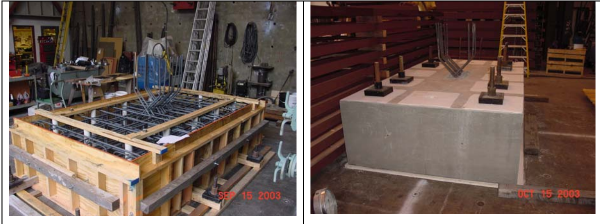
Figure 9.1 Reinforcement and placing of the footing and pin
