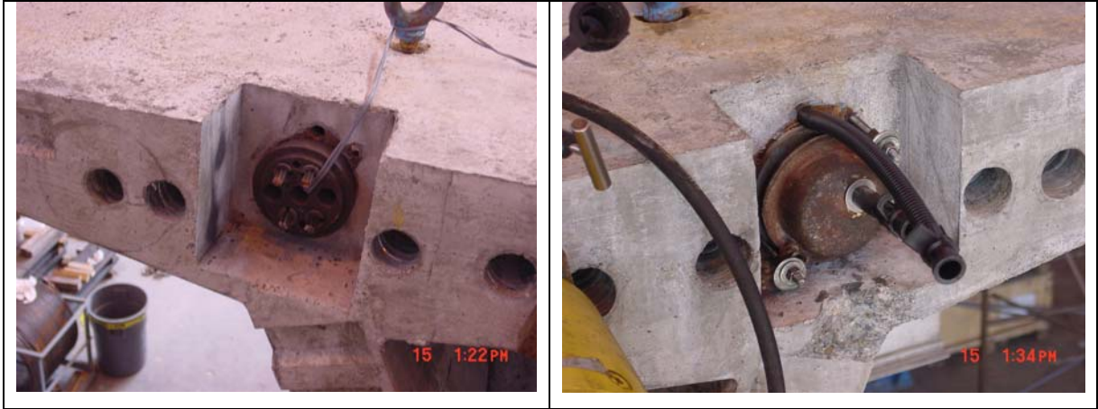
Figure 9.19 Cutting off tendon tails and placement of grout caps
