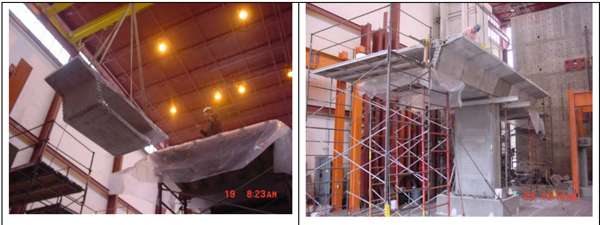
Figure 9.20 2 nd pair of segments installed
