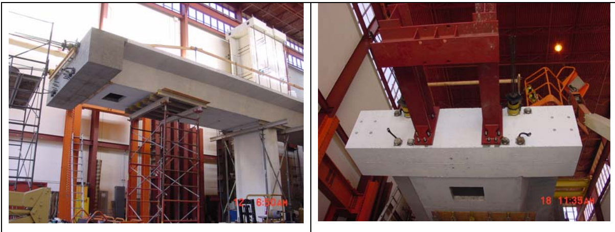
Figure 9.22 Placement of end blocks and fixtures
