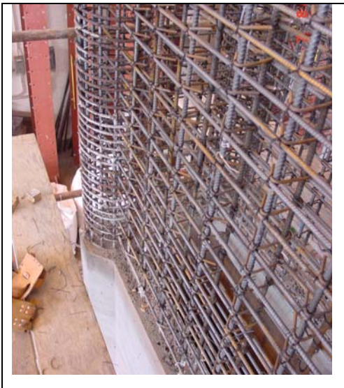
Figure 9.4 View of wall reinforcement in column
