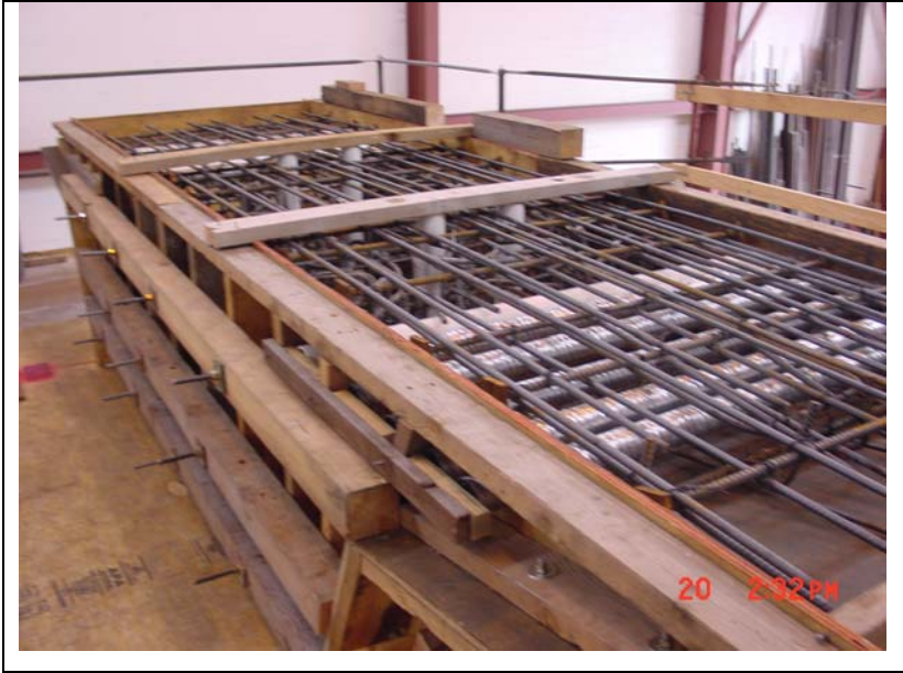
Figure 9.7 Pier segment reinforcement
