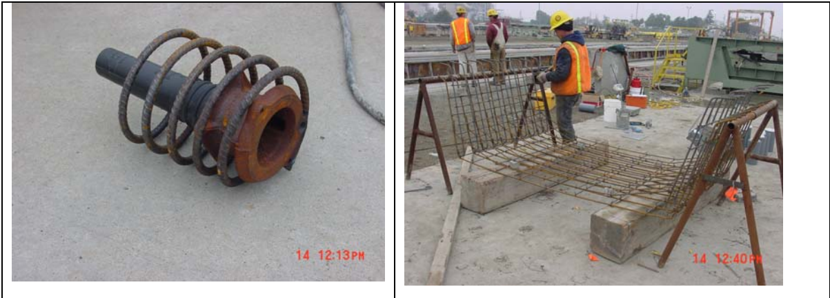
Figure 9.8 Tendon anchor and bottom of superstructure reinforcement cage
