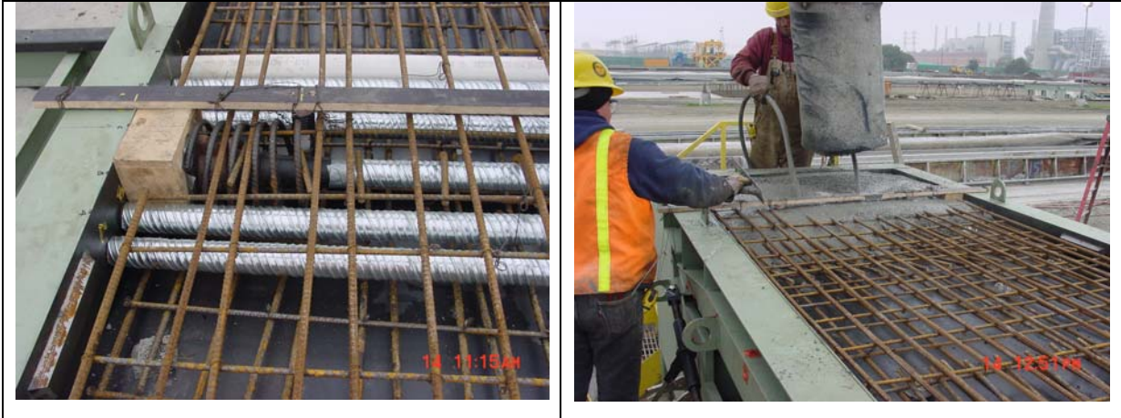
Figure 9.10 Tendons and reinforcement in segment
