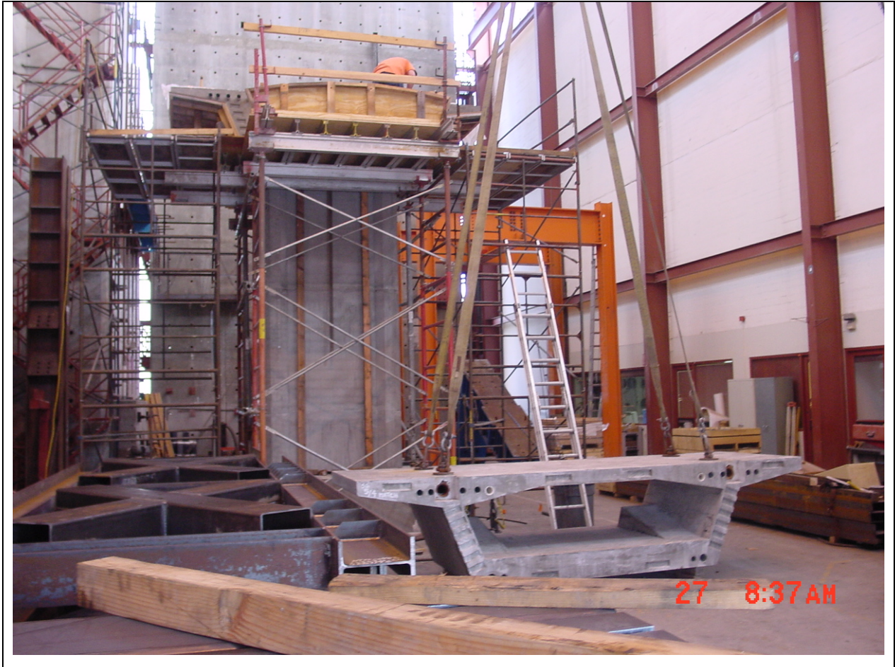
Figure 9.13 Placement of 1 st pair of segments
