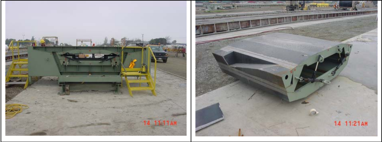
Figure 9.9 Steel forms used for casting superstructure segments, interchangeable inner form
