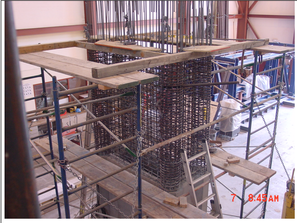
Figure 9.5 Column during construction prior to pouring top portion
