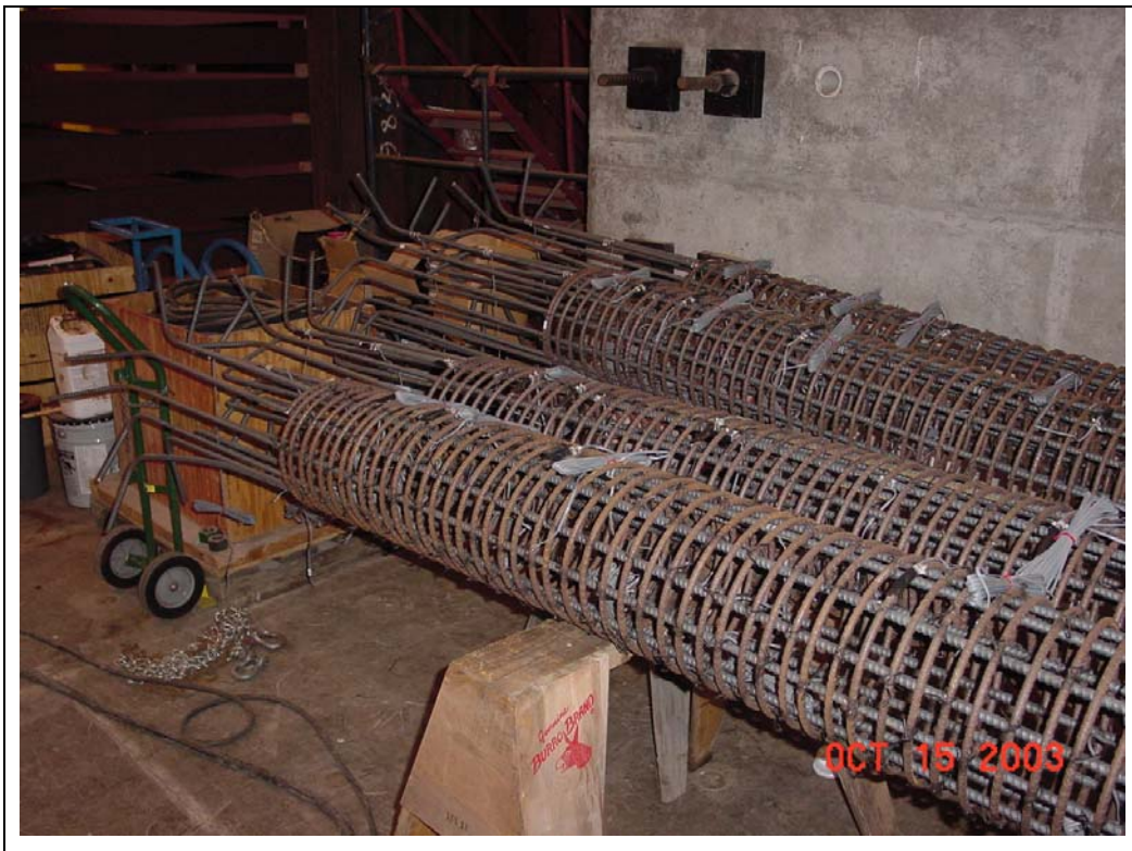
Figure 9.2 Corner spirals with gauges in place
