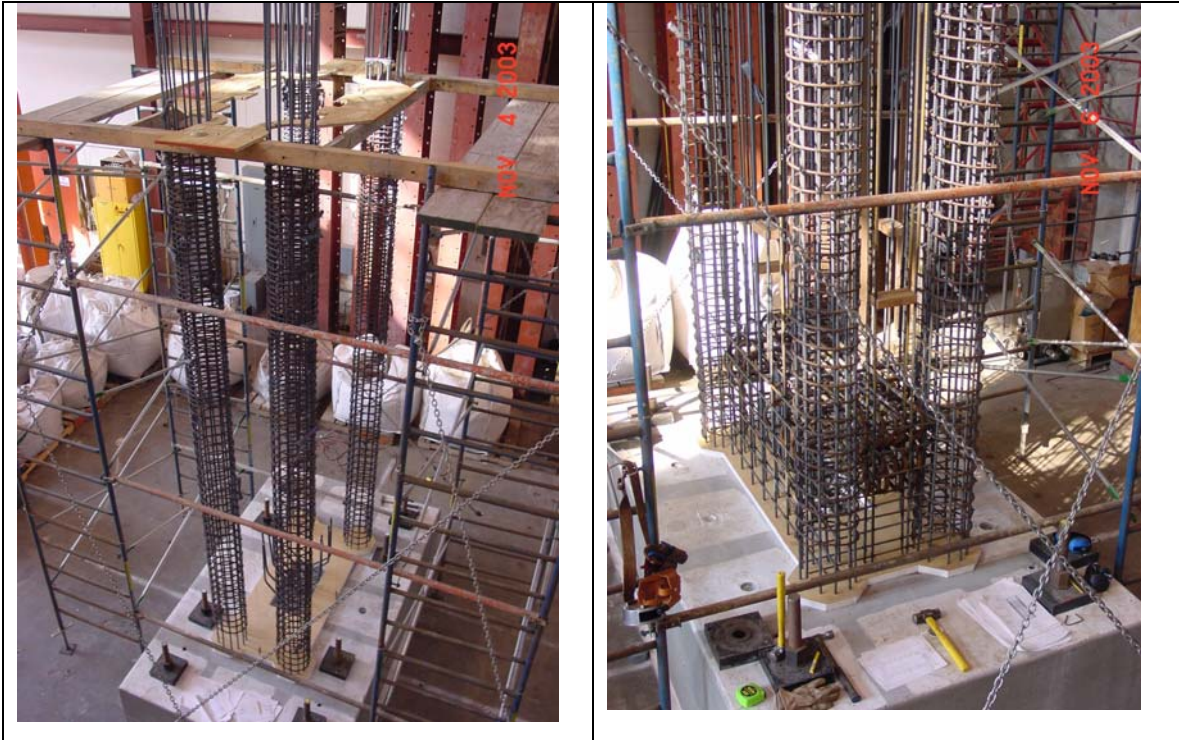
Figure 9.3 Placement of corner spirals and bottom of column reinforcement
