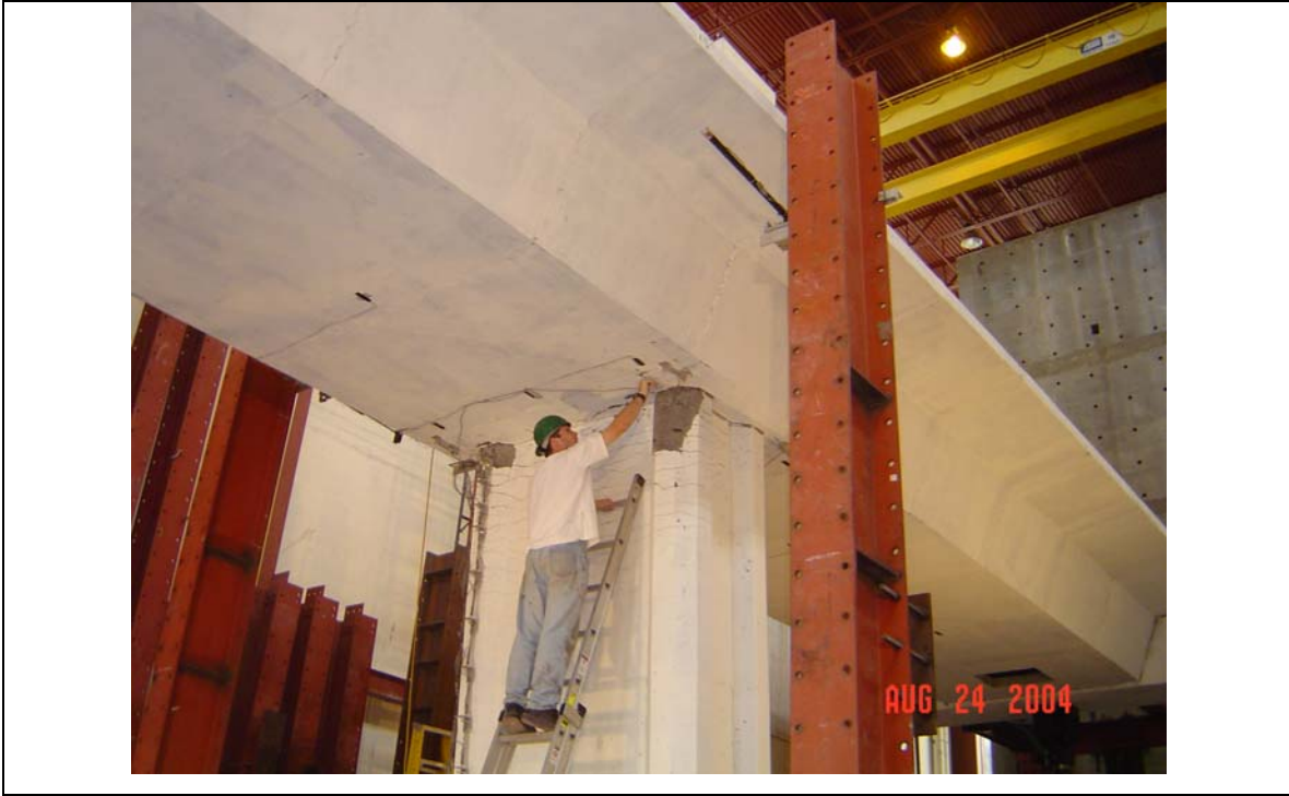
Figure 9.24 Damaged test unit after final testing cycles
