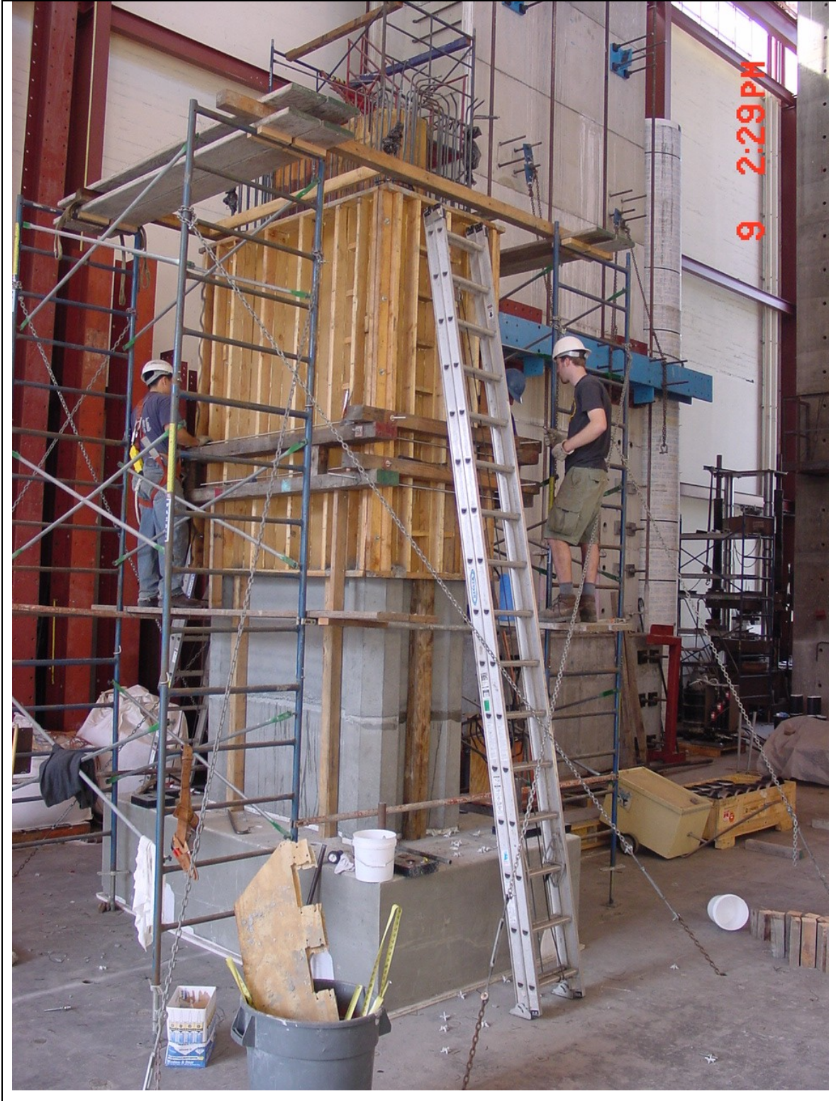
Figure 9.6 Placing forms for pouring top of column
