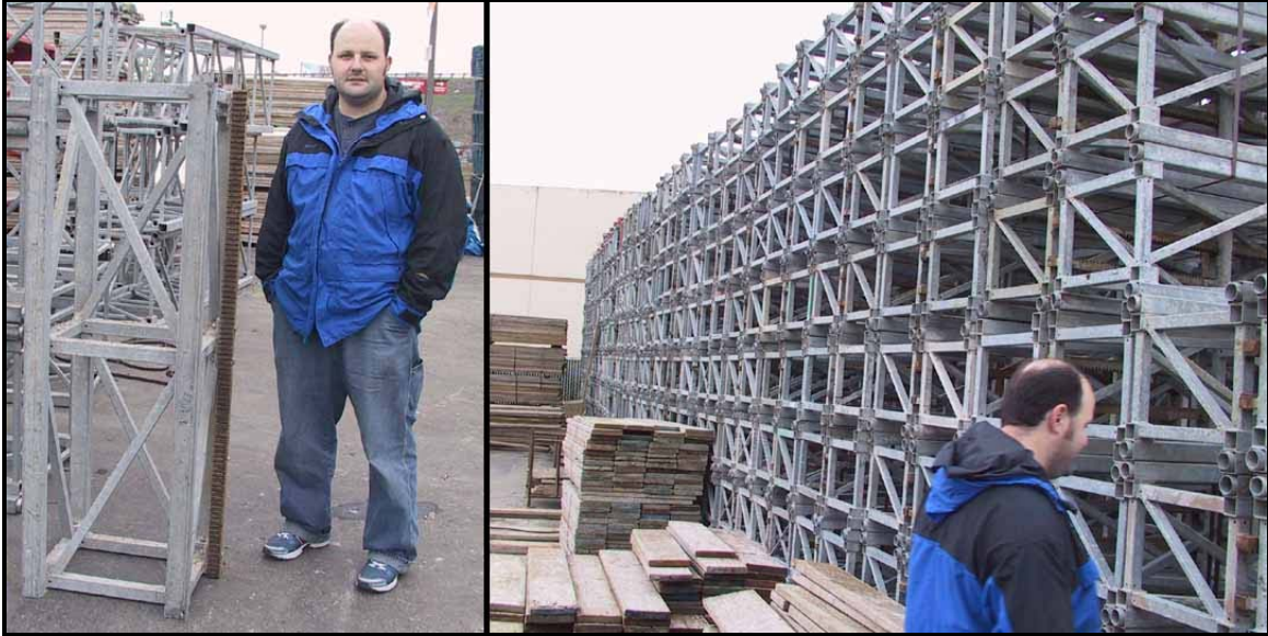
FIGURE 11-A8, INDIVIDUAL SCAFFOLDING PIECE
