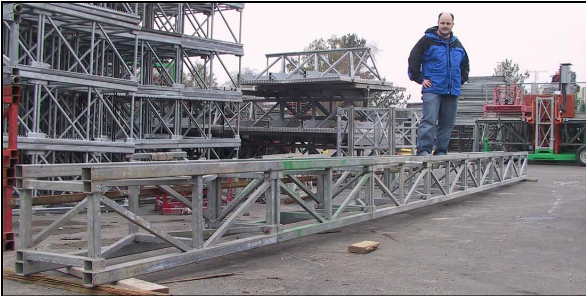
FIGURE 9-A8, MATT STANDING AT CENTER OF SCAFFOLDING SPAN
