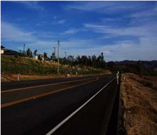
a) High Quality Longitudinal Joint
