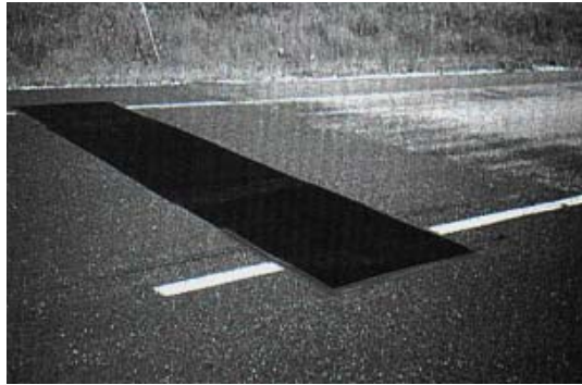
f) Starting Transverse Joints on Roofing Felt Produces Clean Joints
