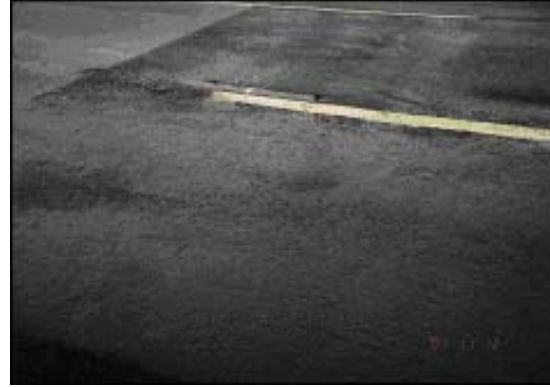
b) Low Quality Transverse Joint
