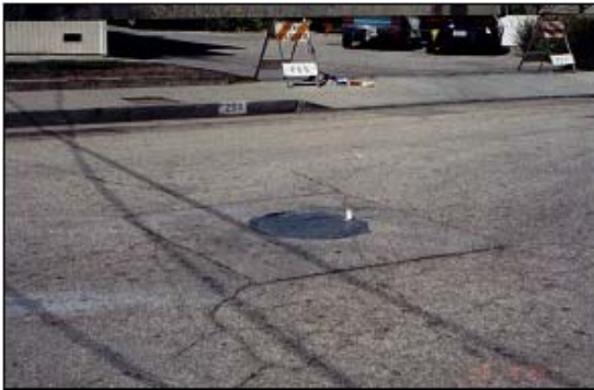
c) Cover Utilities with Kraft Paper
