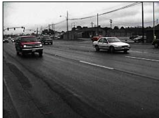
b) Poor Quality Edges and Shoulder
