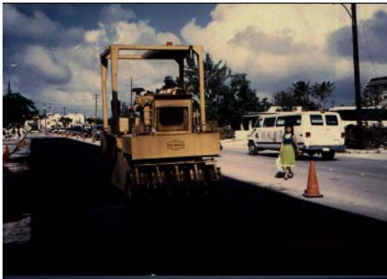
Figure 25: Rolling a Slurry Surfacing
