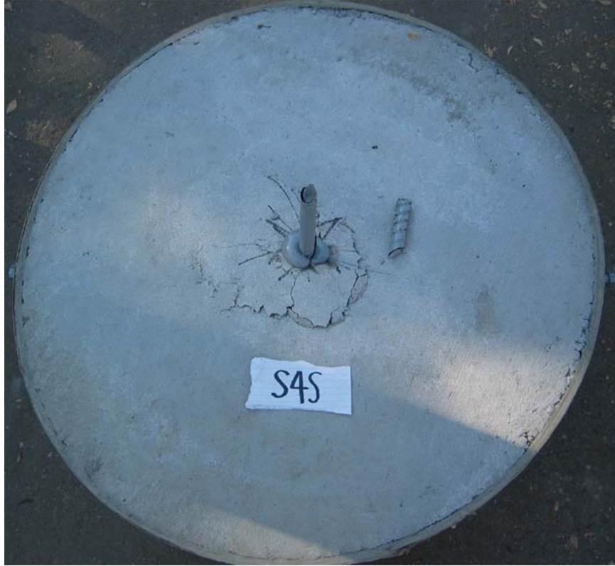
Figure A-5: Typical Rebar Failure
