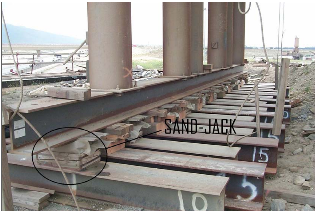
Figure 1.1: Sand-Jacks in use.
