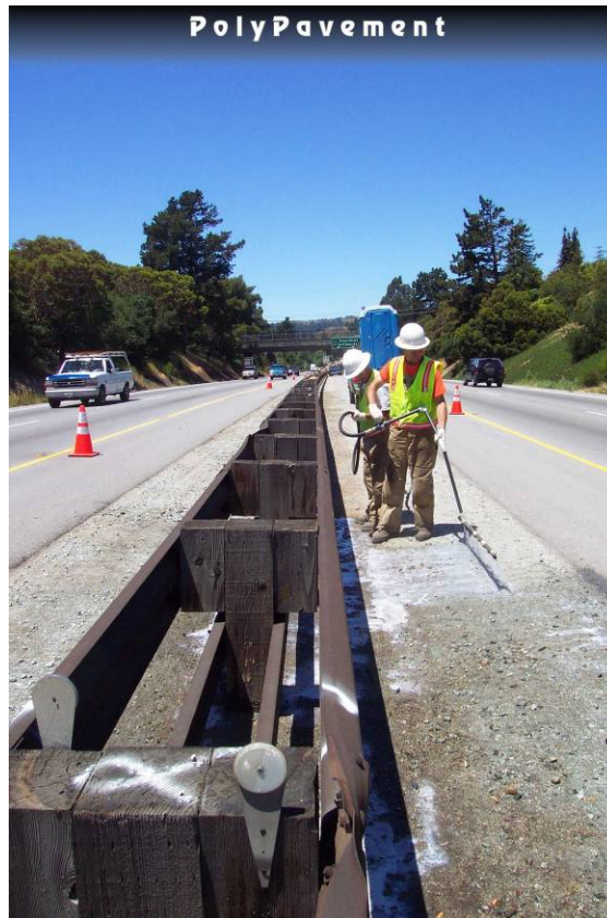
Figure 2.1 Caltrans workers applying PolyPavement weed barrier
