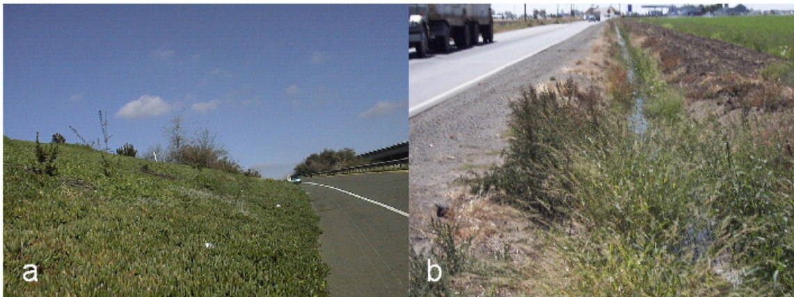
Figure 4.3 Shoulder vegetation along an incline (a) and in a culvert (b).
