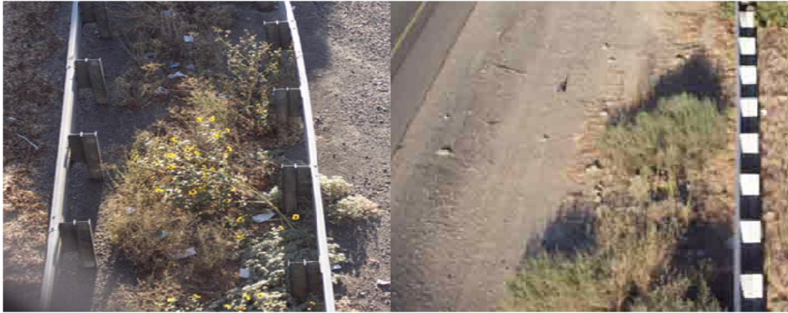
Figure 4.2 Vegetation and debris in between and around guard rails.
