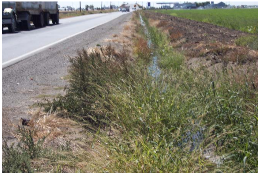
Figure 1.5 V-type Ditch With Irrigation Water
