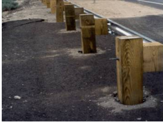
Figure 2.11 Asphalt concrete hardscape
