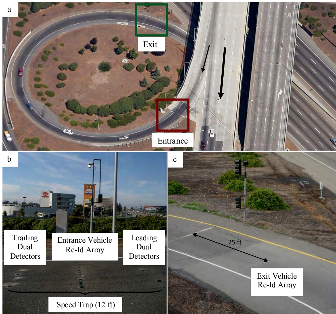
FIGURE 2 (a) Hegenberger on-ramp entrance and exit. (b) Vehicle detection system installation at the entrance of the ramp. (c) Sensor array installation at the exit of the ramp.
