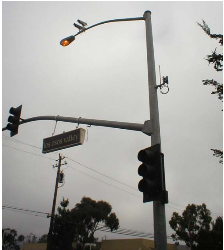
Figure 3. Components of Iteris Vantage (standard color camera) installation at Los Osos Valley Road and Madonna Road Test site: North-facing video camera (day and dusk), overall intersection view.
