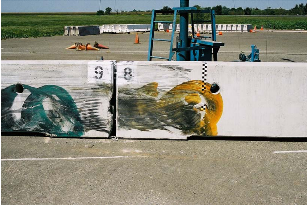
Figure 2-13 – Barrier Damage near the Impact Point
