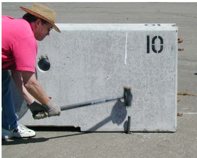
Figure 2-2 – Stake Installation
