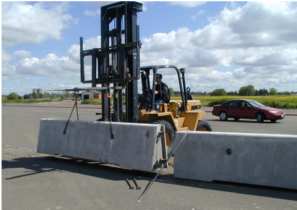
Figure 2-1 – Barrier Placement
