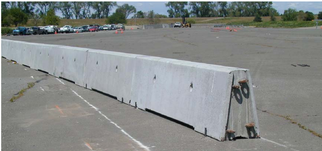
Figure 2-4 – Backside of Completed Barrier with Stakes
