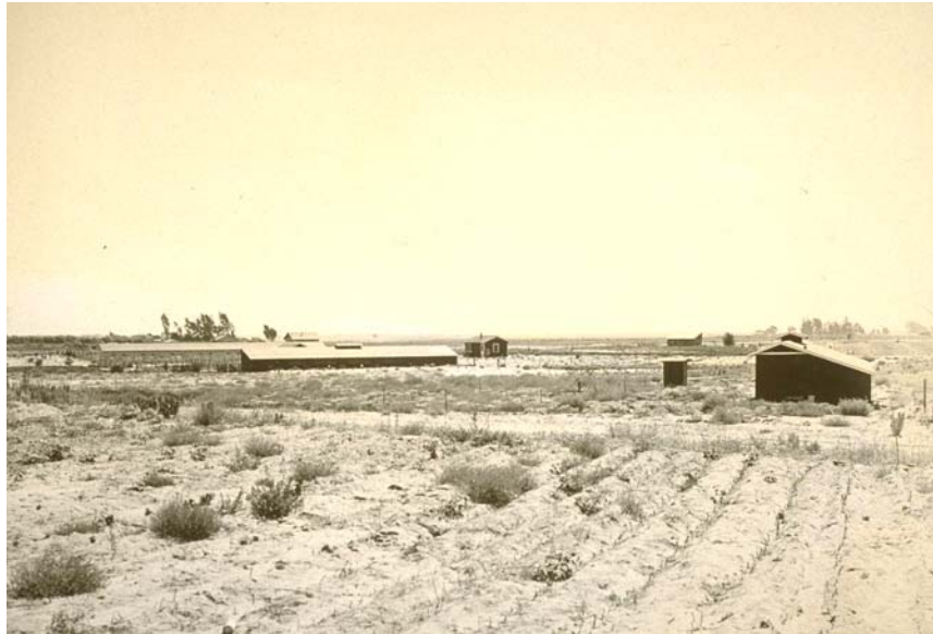
Figure 88: Poultry farm, San Joaquin Valley, circa 1910. Note the long rectangular wood-frame sheds with ventilation stacked gables atop the roof (structures left of photo). Generally poultry sheds were placed far enough from the residence (far right of photo) to avoid the odor associated with the operations (U.C. Berkeley, Bancroft Library).
