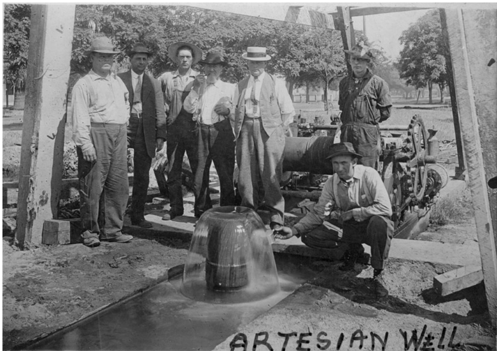
Figure 97: Artesian well near Lemoore, California, circa 1915. Note the concrete derrick above the well (San Joaquin Valley Library System).
