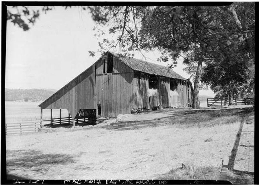
Figure 80: California "bank barn" Mother Lode, Felix, Calaveras County, 1936. Note the stacked rock wall that forms an interior wall and supports the footings for the barn on the upper bank. The lower side of the barn is used for livestock formed by an open-sided shed. (HABS photo, Library of Congress).
