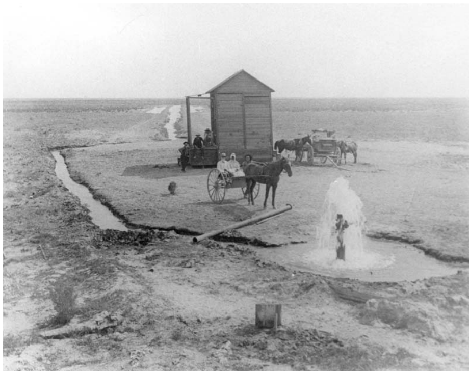
Figure 96: Circa 1880s artesian well, Bakersfield. The wood-frame building in the background probably housed a water storage tank (San Joaquin Valley Library System).
