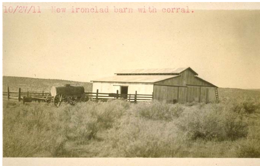
Figure 82: Sheep barn clad with corrugated iron sheeting, 1911. The use of galvanized iron panel siding was that it cut down on maintenance, and provided sheer wall strength.. Note the low profile of the barn and the barn's centrally located stacked gable that serves as ventilation. The corral adjacent to the barn was used to secure ewes and sheep during shearing season and from predators, such as coyotes (U.C. Berkeley, Bancroft Library).
