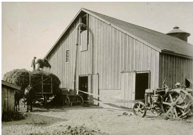
Figure 83: Typical California wood or stick-frame dairy barn at the F.E. Baxter Ranch, Durham, California, circa 1920. Note the board and batten siding, poured concrete perimeter or stem wall foundation, and lack of any stacked ventilation gable. The pop-out side windows, sidewall vent and large bay doors may have been adequate to ventilate the building during the hot summer months. This barn may have a poured concrete floor for improved sanitation. Other features include the silo on the opposing side, and feed loft. In this photograph a traction engine is being used to force-feed or grain through a centrifugal device up a pipe and into the loft (U.C. Berkeley, Bancroft Library).
