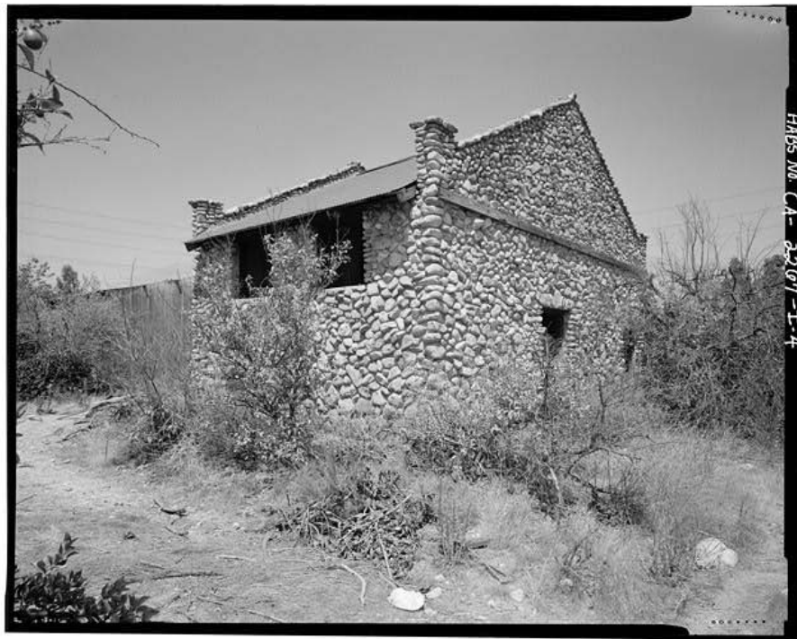
Figure 93: Pitzer Ranch Barn, Claremont, Los Angeles County, n.d. In this case the structure is built of concrete and the walls are clad with cobbles obtained locally (HABS photo, Library of Congress)
