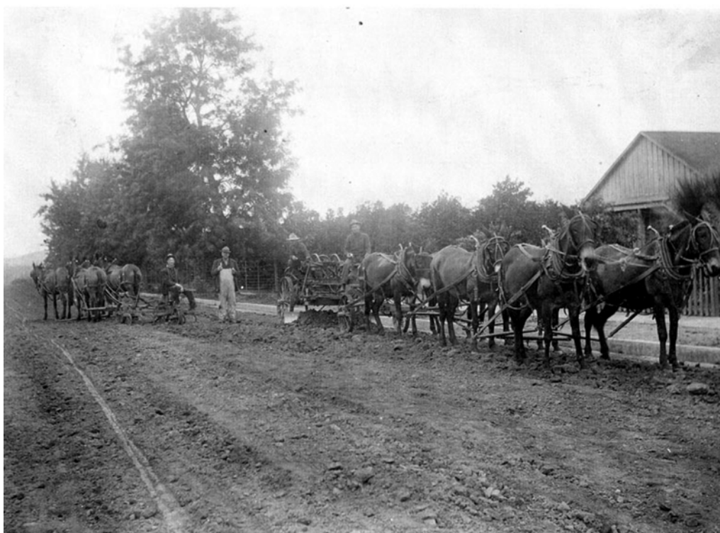
Figure 47: Road building with Fresno Scrapers in Kings County, ca. 1915 ( The San Joaquin Valley Digitization Project, Kings County Library, CA, San Joaquin Valley & Sierra Foothills Photo Heritage, kia0116, San Joaquin Valley Library System, Fresno, California ).
