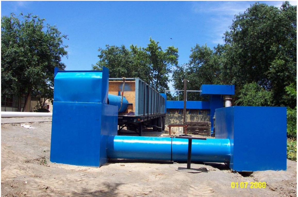
Fig. 2.12: Downstream receiving tanks.
