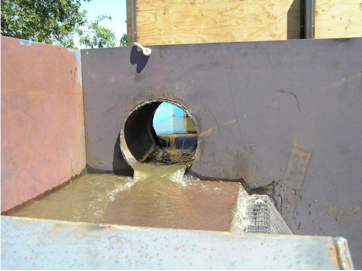
Fig. 6.8: View inside inflow pipe for Q=0.94 cfs.
