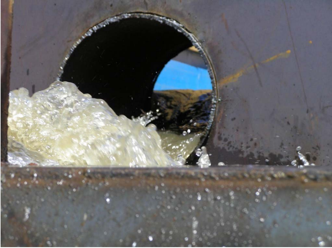
Fig. 6.14: Conditions inside inflow pipe at Q=2.7 cfs.
