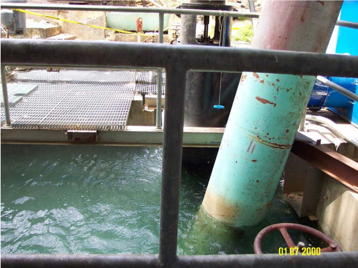
Fig. 2.3a: Sump, pump and overflow return.
