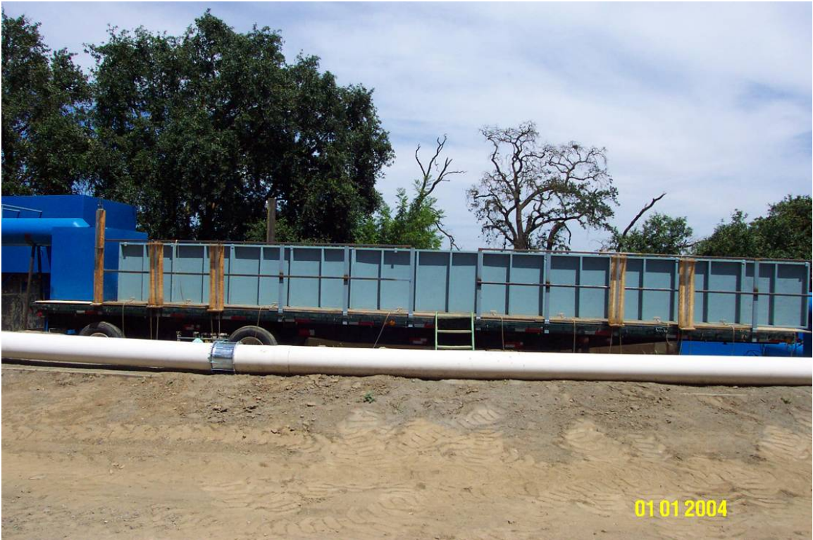
Fig. 2.9: Vault on flat trailer bed.
