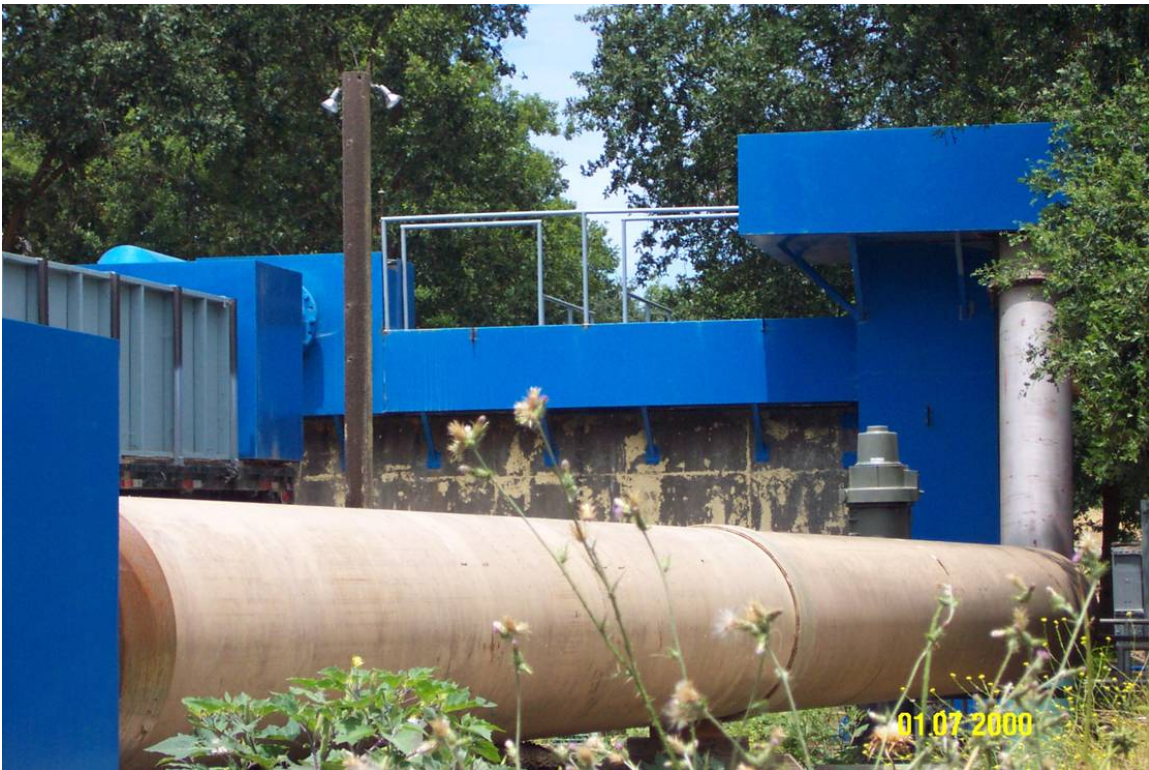
Fig. 2.14: 3' diameter return pipe to sump.
