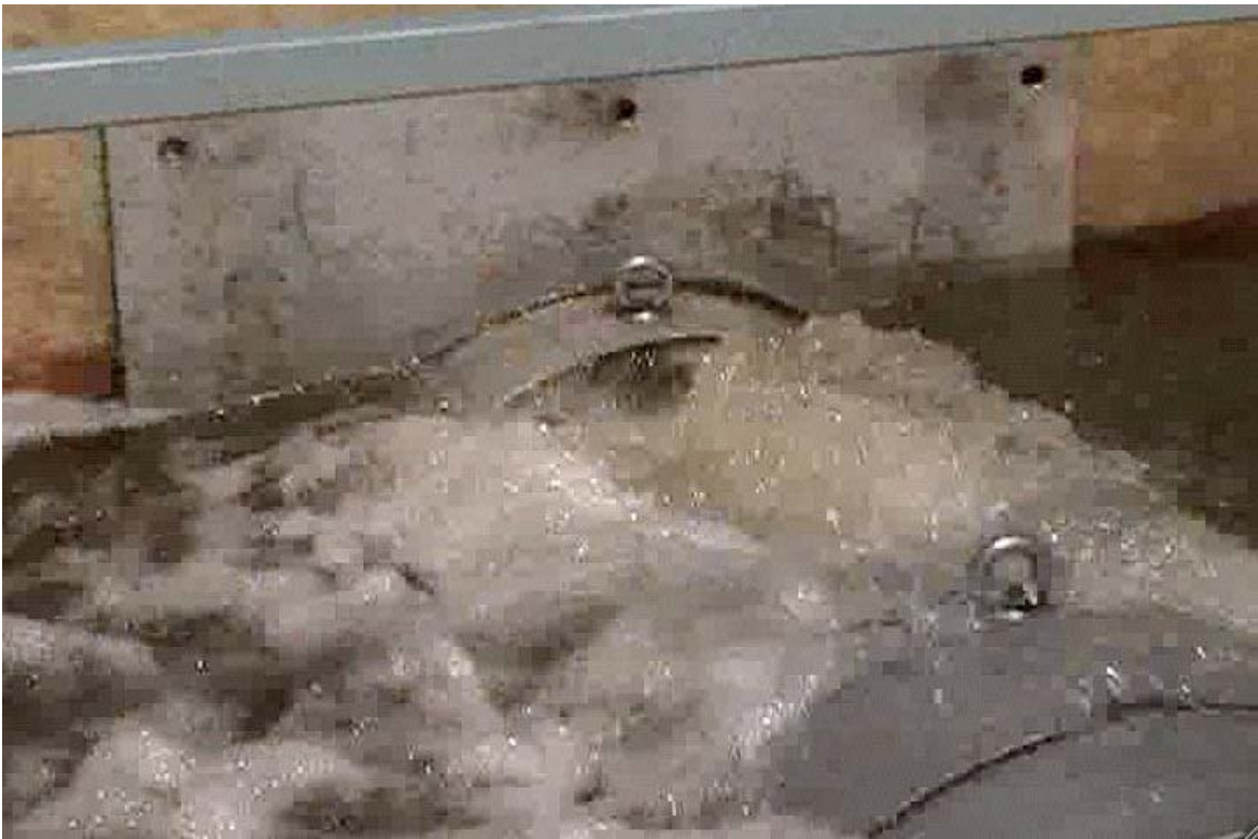
Fig. 4.58: Close-up of overflow
