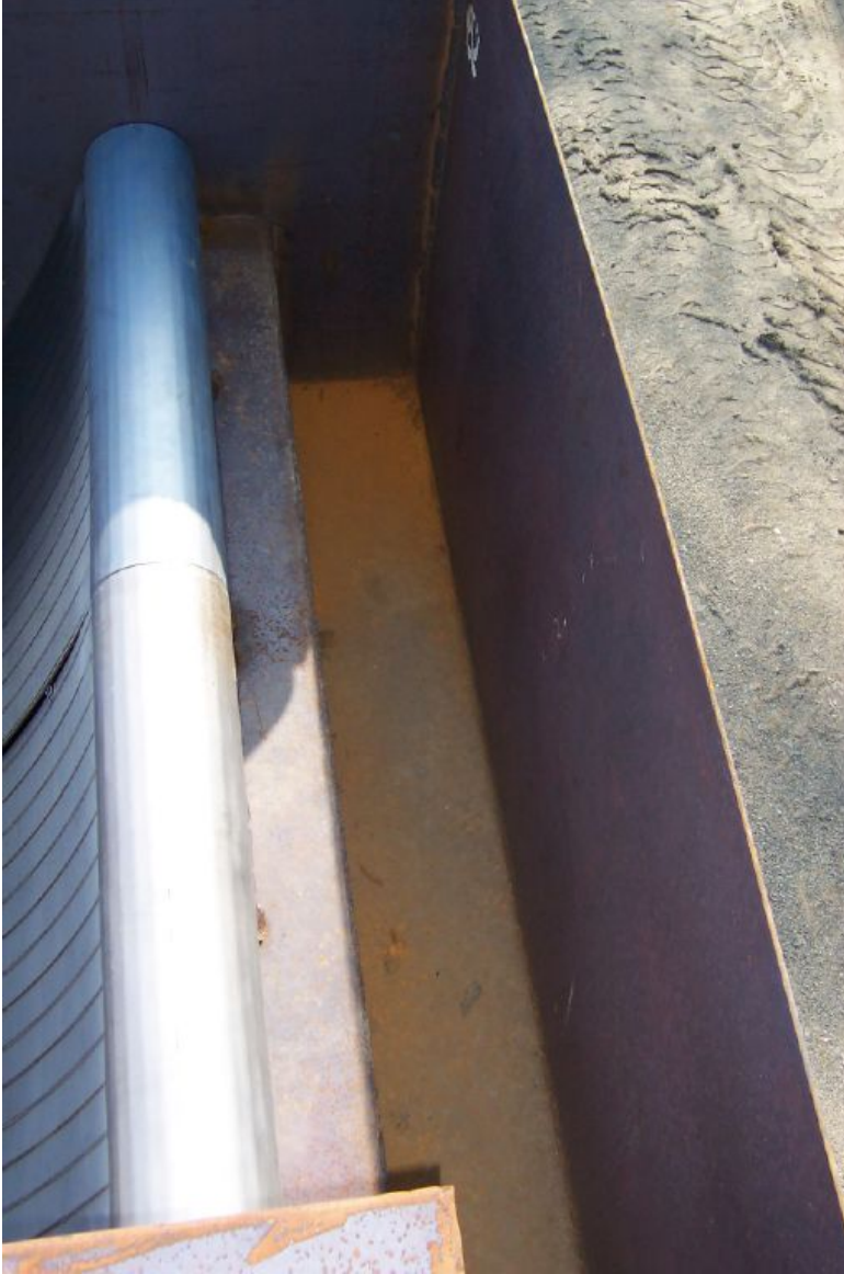
Fig. 5.5: View of the influent trough and solids trap showing the parabolic wedgewire screens in place below the curved weirs.
