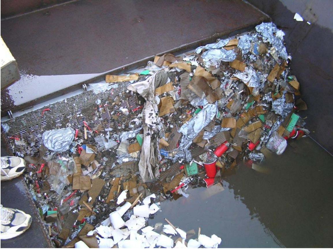
Fig. 6.49: Aftermath of Q=5.5 cfs and 50% loading.
