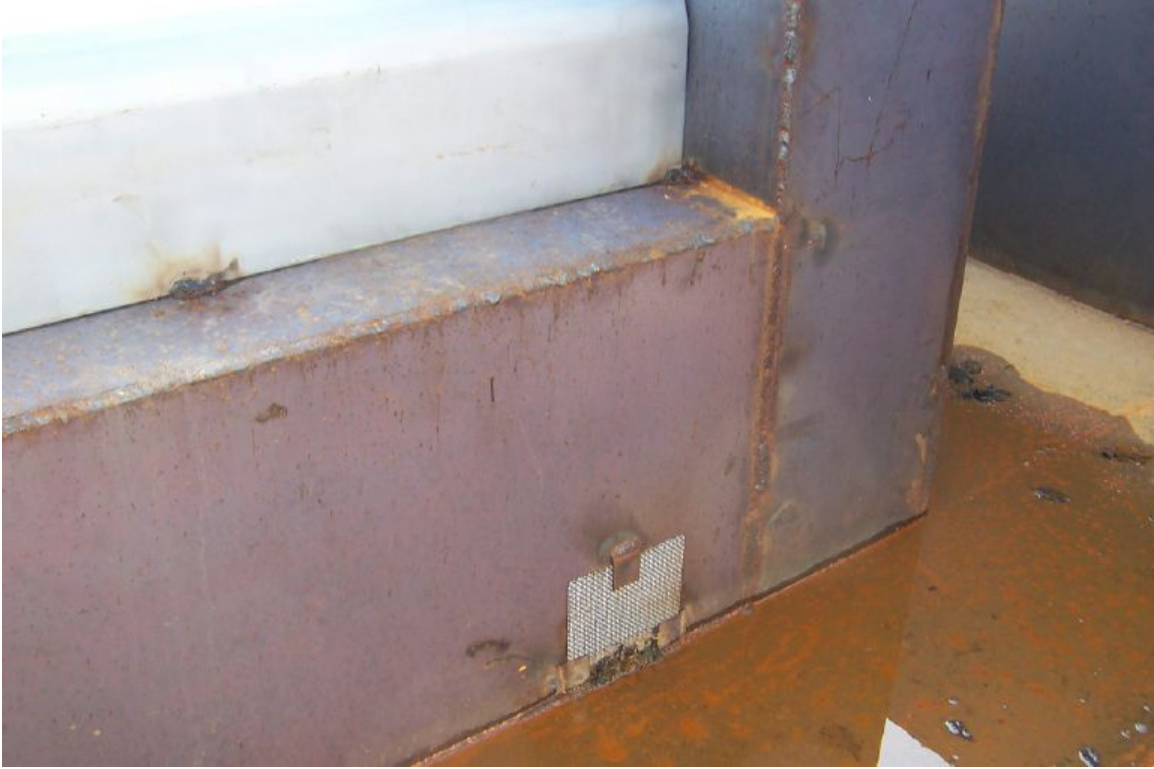
Fig. 5.4: Weep holes used to drain the runoff which accumulates in the influent trough.
