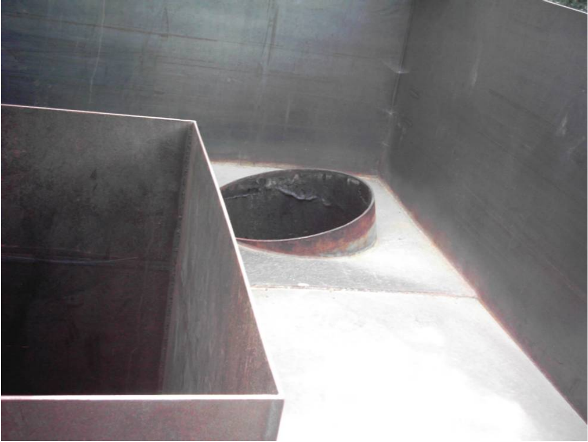
Fig. 2.7: Overspill weir and return to sump.
