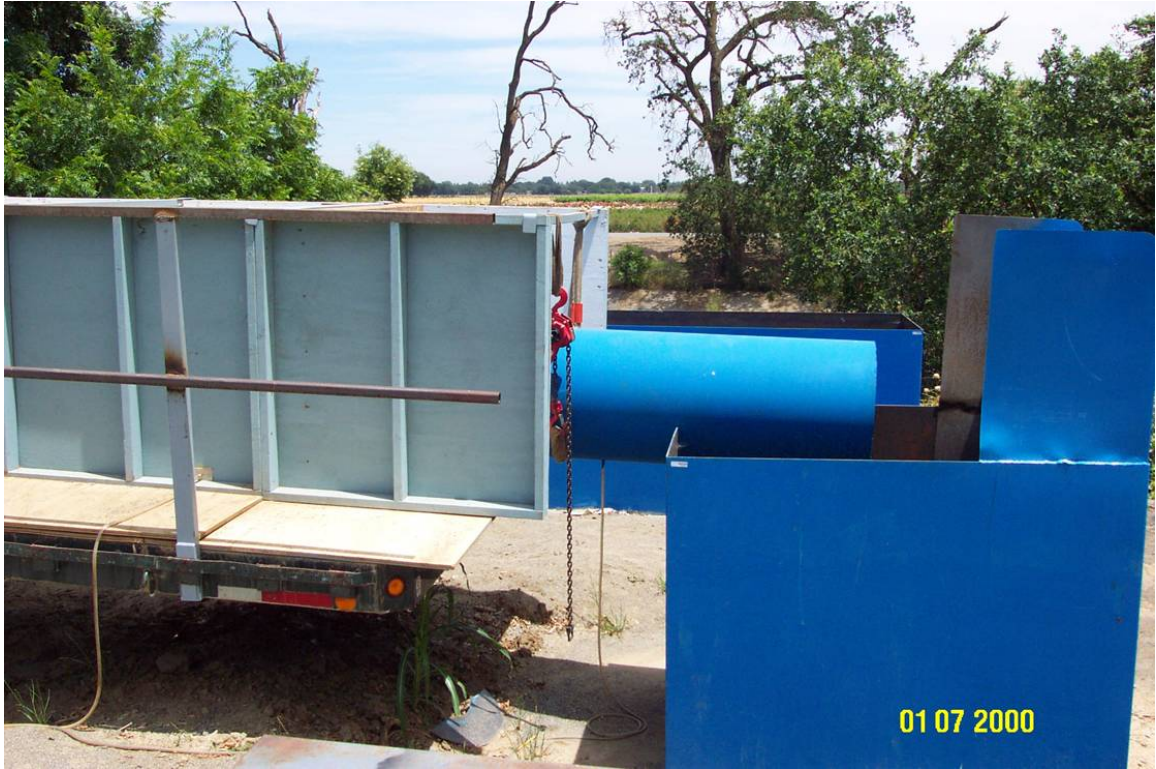
Fig. 2.11: Outfall from vault and downstream receiving tank.
