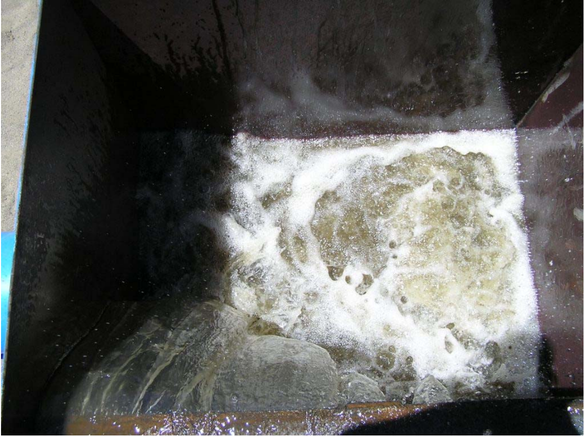
Fig. 6.31: Conditions in exit tank and the spill over of flow from the inflow shelf.
