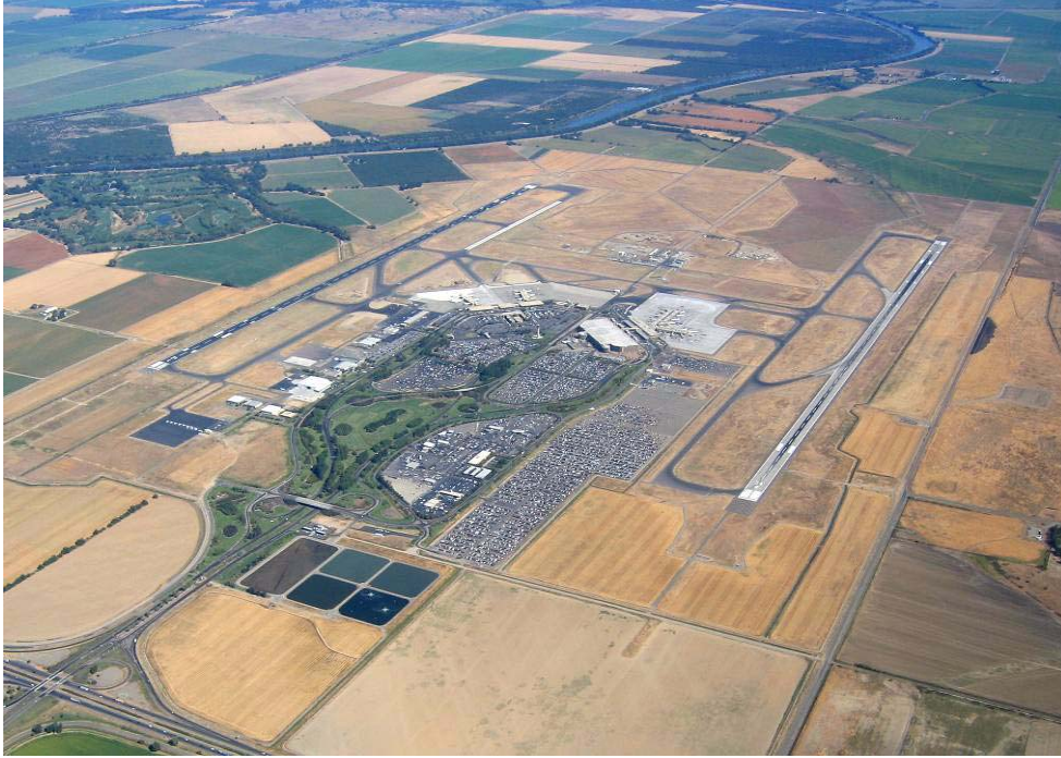
Figure 1 Sacramento International Airport
