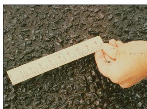
Figure 6: Chip Seal Before and After Fog Seal
