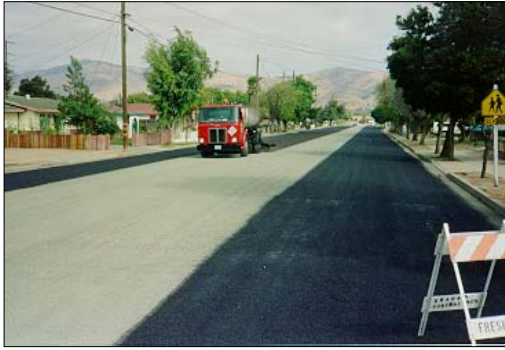
Figure 2: Fog Seal Application
