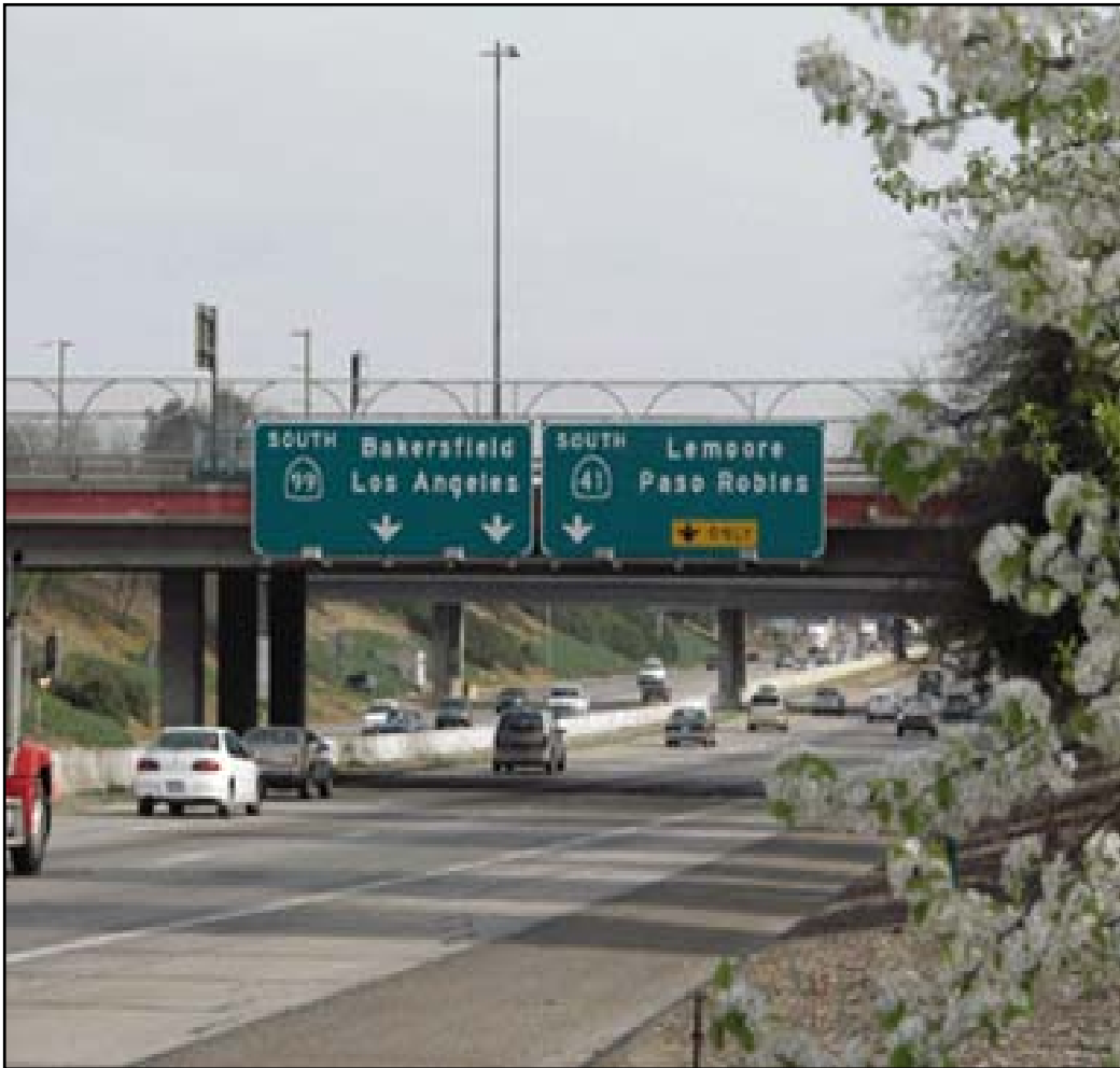
Route 99 in Fresno County
