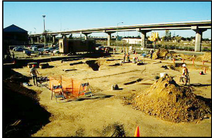
LARGE-SCALE ARCHAEOLOGY on Seventh Street. Archaeologists used a backhoe-loader to expose the surface of a large portion of this city block adjacent to the elevated BART tracks and close to the U.S. Postal Service facility. Here they uncovered building remains, wells, and other features from West Oakland's past.
