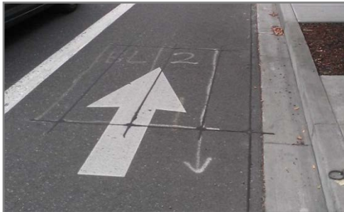
c. Quadrupole Bicycle Loop Detector at 99E and Couch St., Portland, OR
