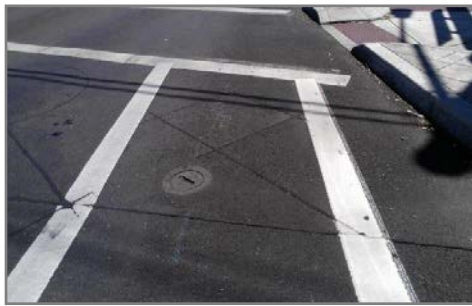
a. Diamond Bicycle Loop Detector at 99W and Hall Boulevard, Tigard, OR
