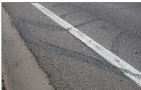
e. Parallelogram Loop Detector Used for Bike Lane Signal Actuation in Boulder, CO
