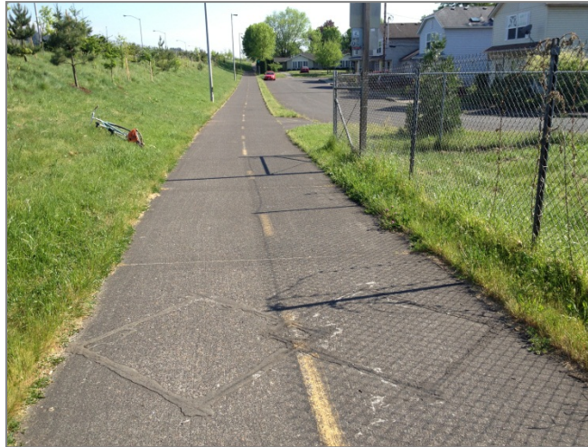
Figure 4.3. I-205 Path Inductive Loops
