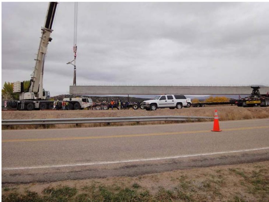
Girders for the replacement structure, N-17-Q arrived at the site on trucks. The span was too wide for a single crane to set the girders so a pair of cranes, one at each end of the structure, positioned the girders. The east end of a girder was lifted from its truck by the crane at the west abutment.
