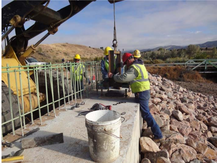
Figure 15 – Setting of Bearings (Note: A special clamping bar was used to lift the bearings.)
