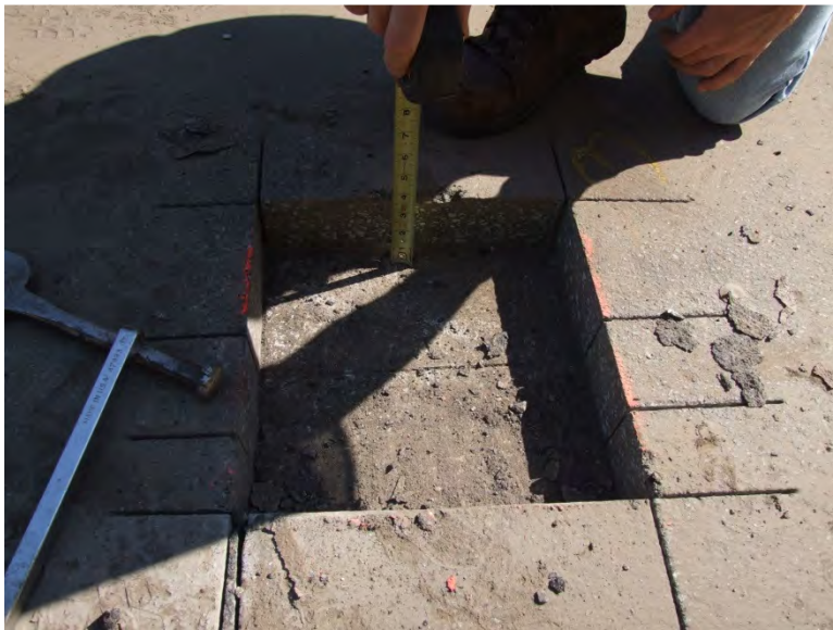
Figure 17. Asphalt Removed at Location 3
