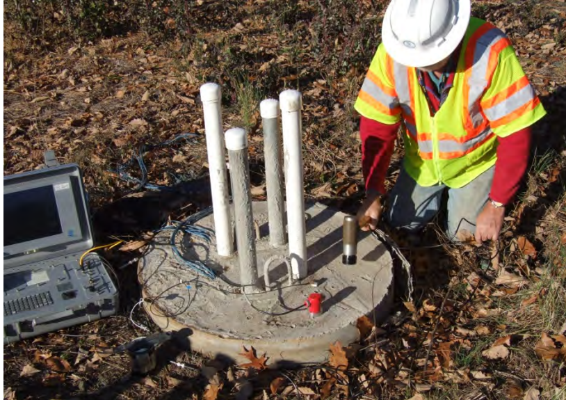
Figure 4. Sonic Echo–Impulse Response Testing at VDOT’s Boyd Tavern Area Headquarters
