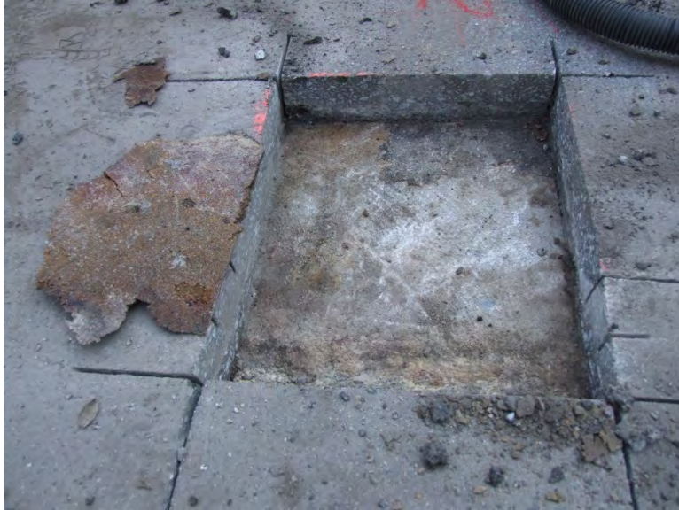
Figure 16. Asphalt Removed at Location 2
