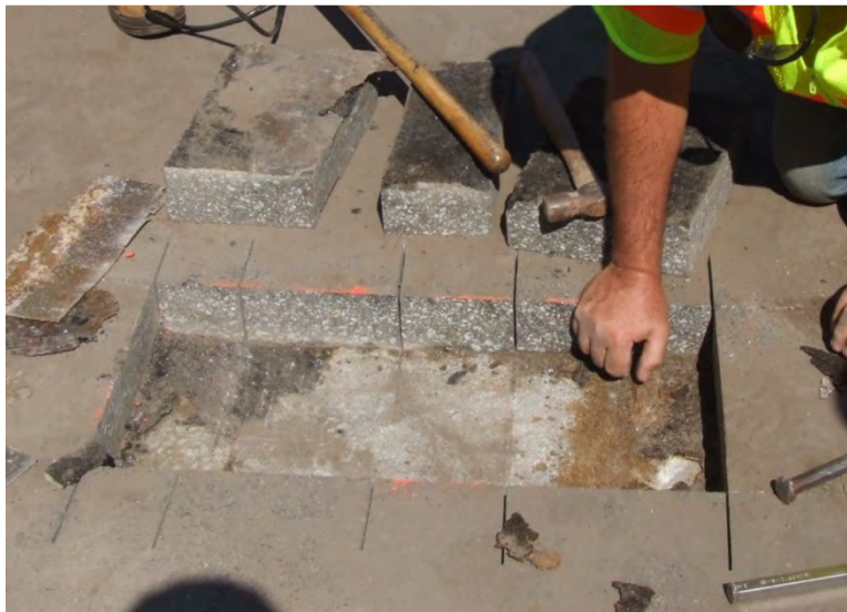
Figure 15. Asphalt Removed at Location 1
