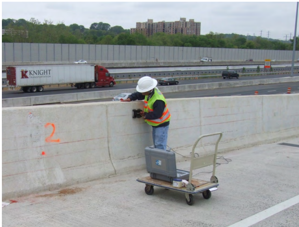
Figure 23. Use of Impact Echo Scanner on Parapet
