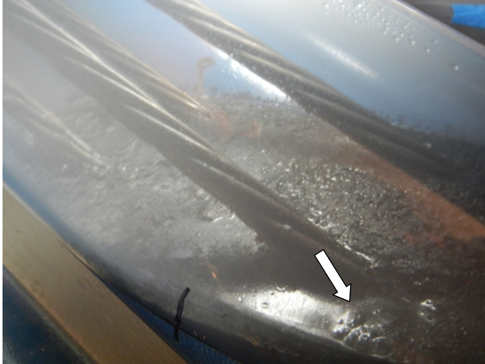
Figure 156. Photo. Void condition of 0 percent chloride specimen.
