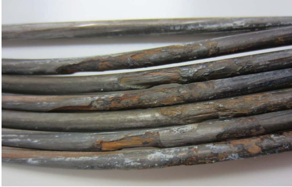
Figure 217. Photo. As-extracted condition of a stressed segment passed through the contaminated void/grout interface of 0 percent chloride multi-strand specimen.
