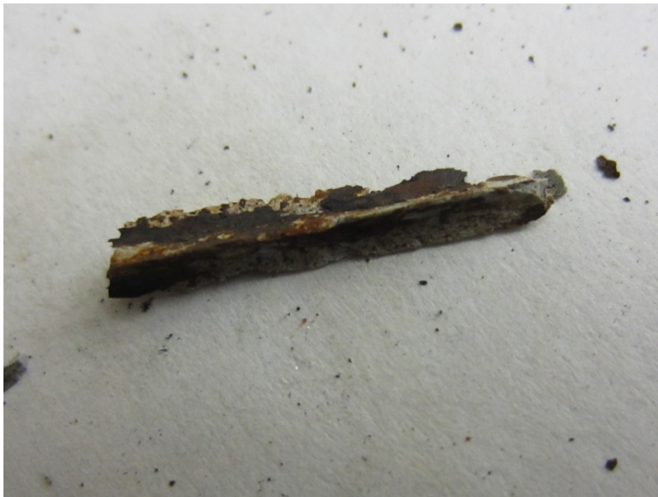
Figure 236. Photo. Heavily rust-stained grout fragment that fell from the strand shown in figure 235.
