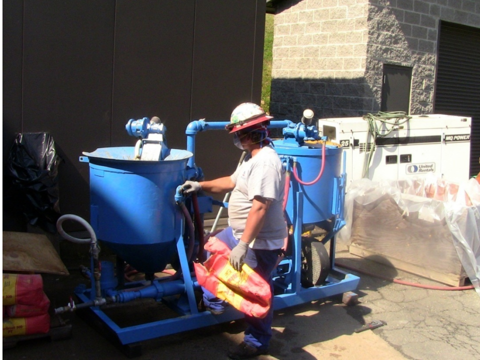
Figure 32. Photo. Grout mixing.
