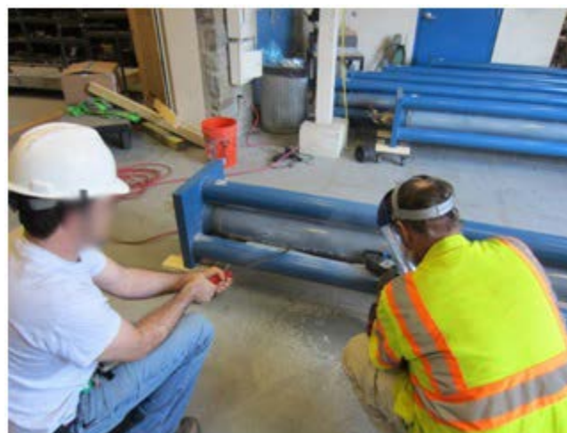
Figure 68. Photo. Cutting the clear duct to expose grout.
