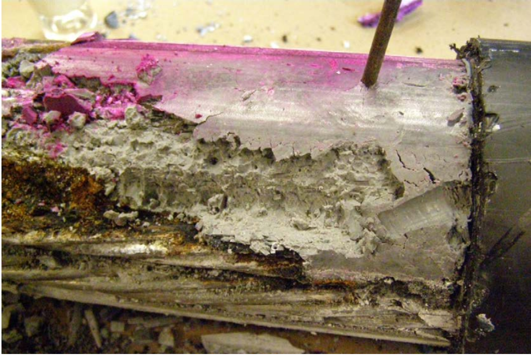
Figure 269. Photo. External PT tendon of Ringling Causeway bridge in Florida. (4)
