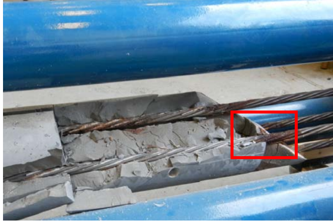
Figure 227. Photo. Severely corroded strand with one broken wire revealed at the void/grout interface of 2.0 percent chloride multi-strand specimen.
