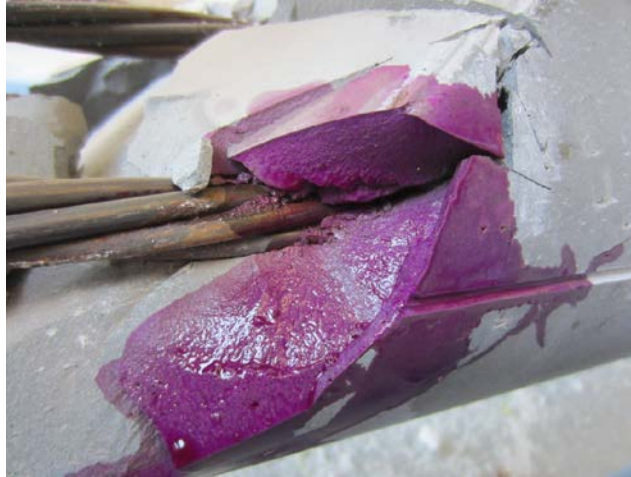
Figure 231. Photo. Carbonation testing results of 0.6 percent chloride multi-strand specimens.
