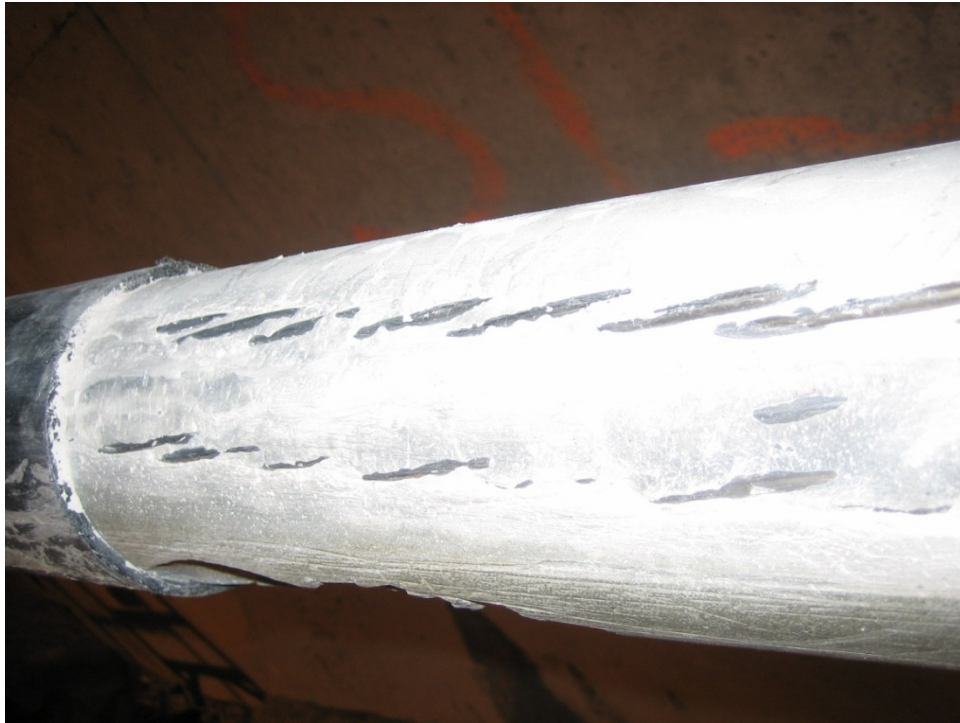
Figure 267. Photo. External PT tendon of Verina-Enon bridge in Virginia.
