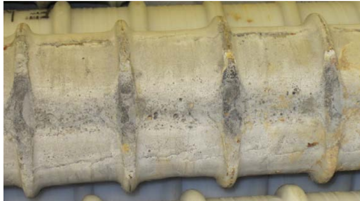
Figure 224. Photo. Defective grout along a bleed channel.
