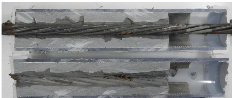
Figure 198. Photo. Stressed single-strand specimen with void and 2.0 percent chloride.
