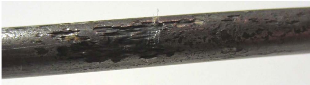
Figure 242. Photo. 0.6 percent chloride multi-strand specimen in the grout (pit depth = 2–14 mil).
