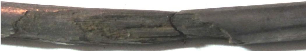
Figure 246. Photo. 0.4 percent chloride multi-strand specimen near the void (pit depth = 2–50 mil).
