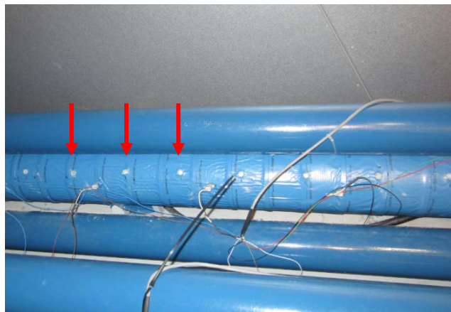
Figure 58. Photo. Drilled multi-strand specimen with 0.8 percent chloride.
