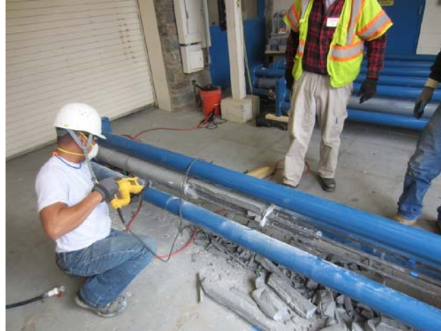
Figure 69. Photo. Chipping grout to expose PT strands.
