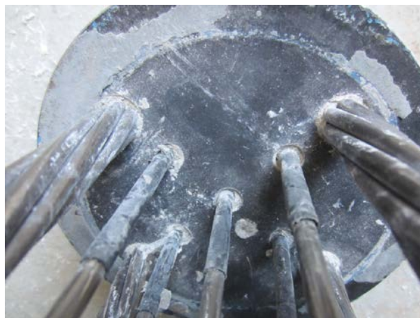
Figure 200. Photo. Exposed interior side of lower anchor plate.
