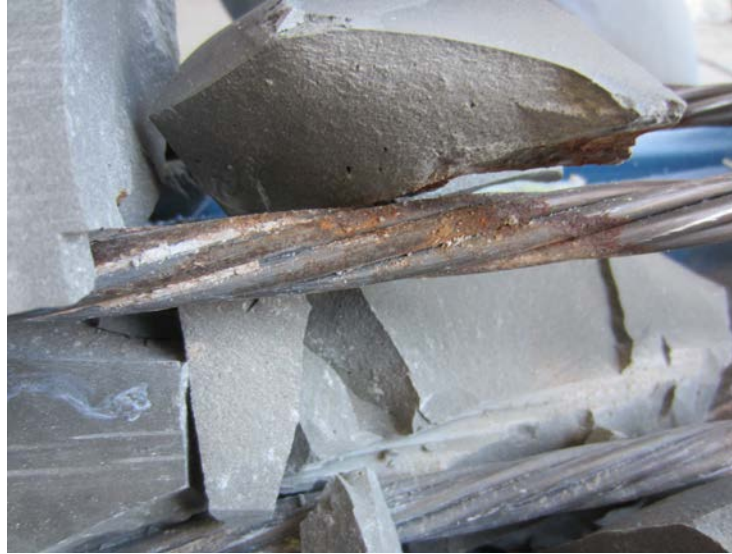
Figure 211. Photo. Exposed strand at the interface of 0.8 percent chloride multi-strand specimen.
