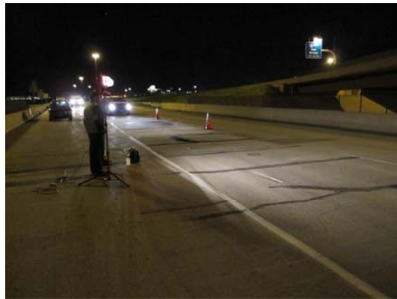
Fig 3.3 One shoulder lane and two traffic lanes of Bridge E-17-QM
