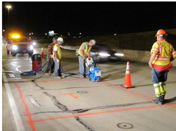
Fig 3.5 Cleaning the deck surface
