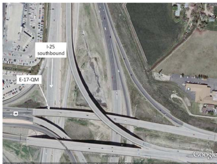
Fig 3.1 Bird's eye view on Bridge E-17-QM
