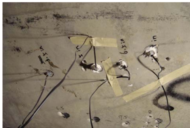
Fig 3.14 Integrated sensors installed in the deck.
