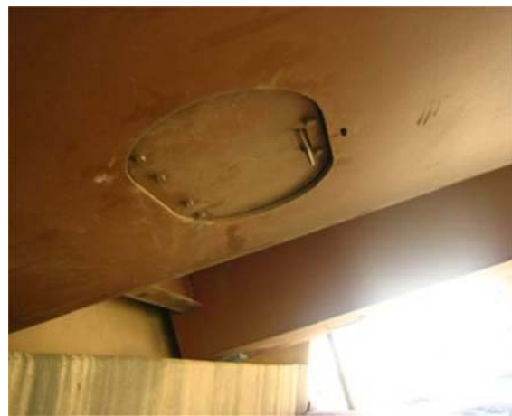
Fig 3.4 A hatch beneath the bridge for accessing the steel box girder
