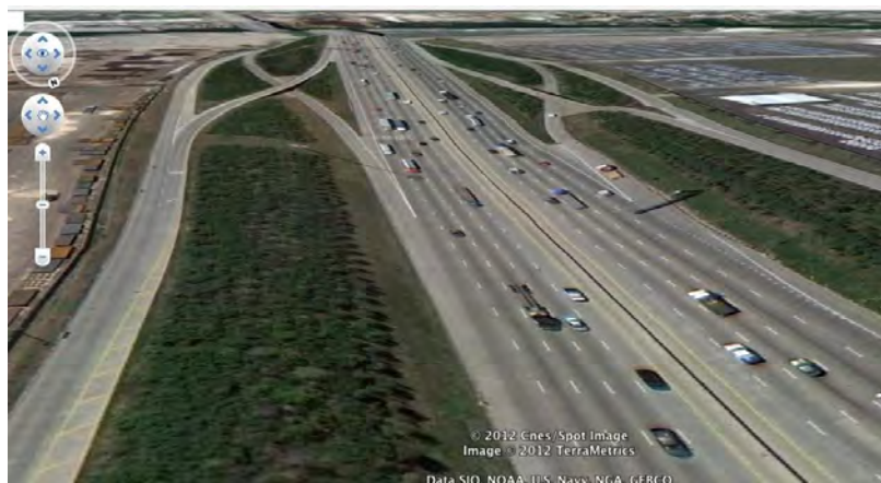
Figure 3.2 Google Earth Image of IH 610 Work Zone Area.
