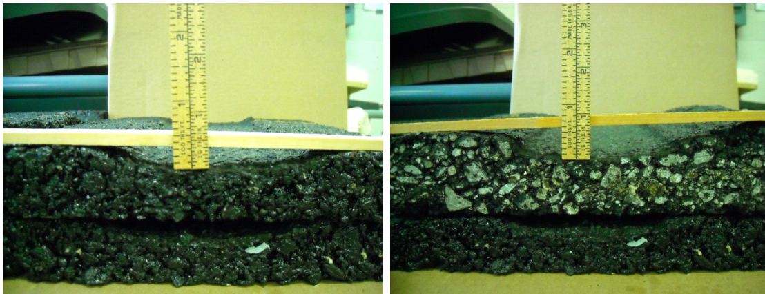
Figure 11. Difference in Rutting Between SM-9.5A HR (left) and SM-12.5D HR (right) Mixtures. Excessive heaving can be observed in the SM-12.5D mixture
