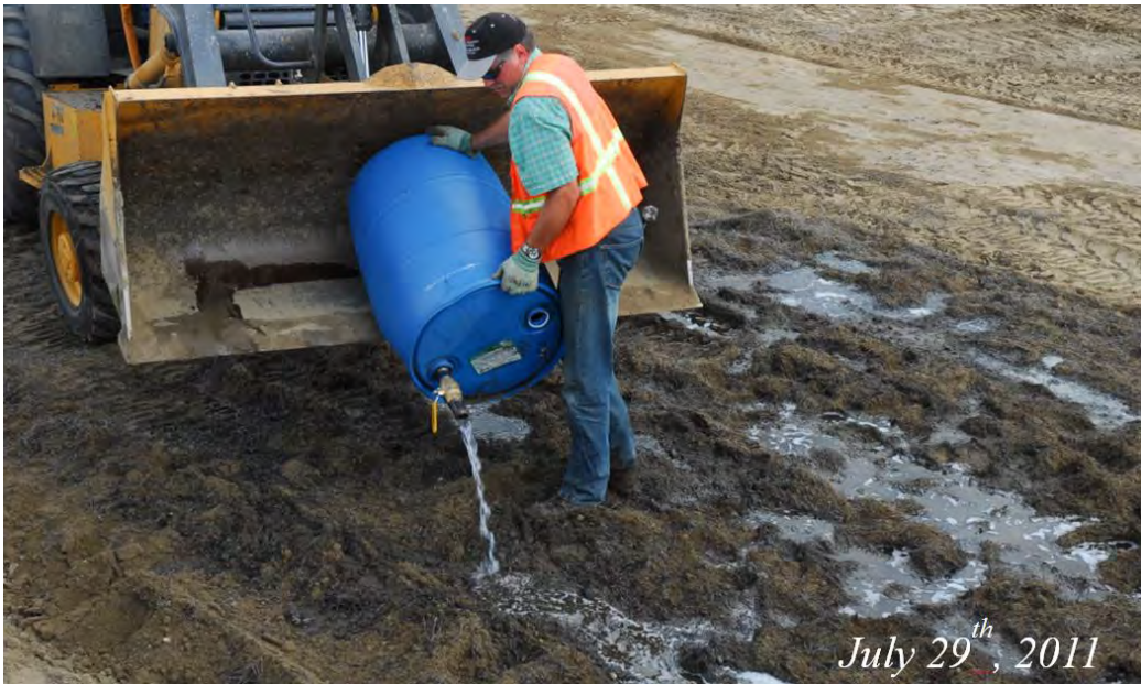
Fig. 3-9: Addition of liquid additive
