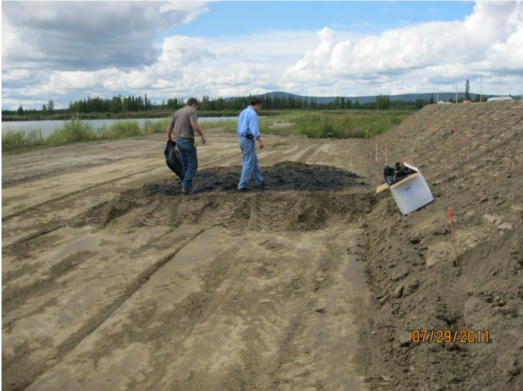
Fig. 3-10: Geofibers added to stockpiled soil
