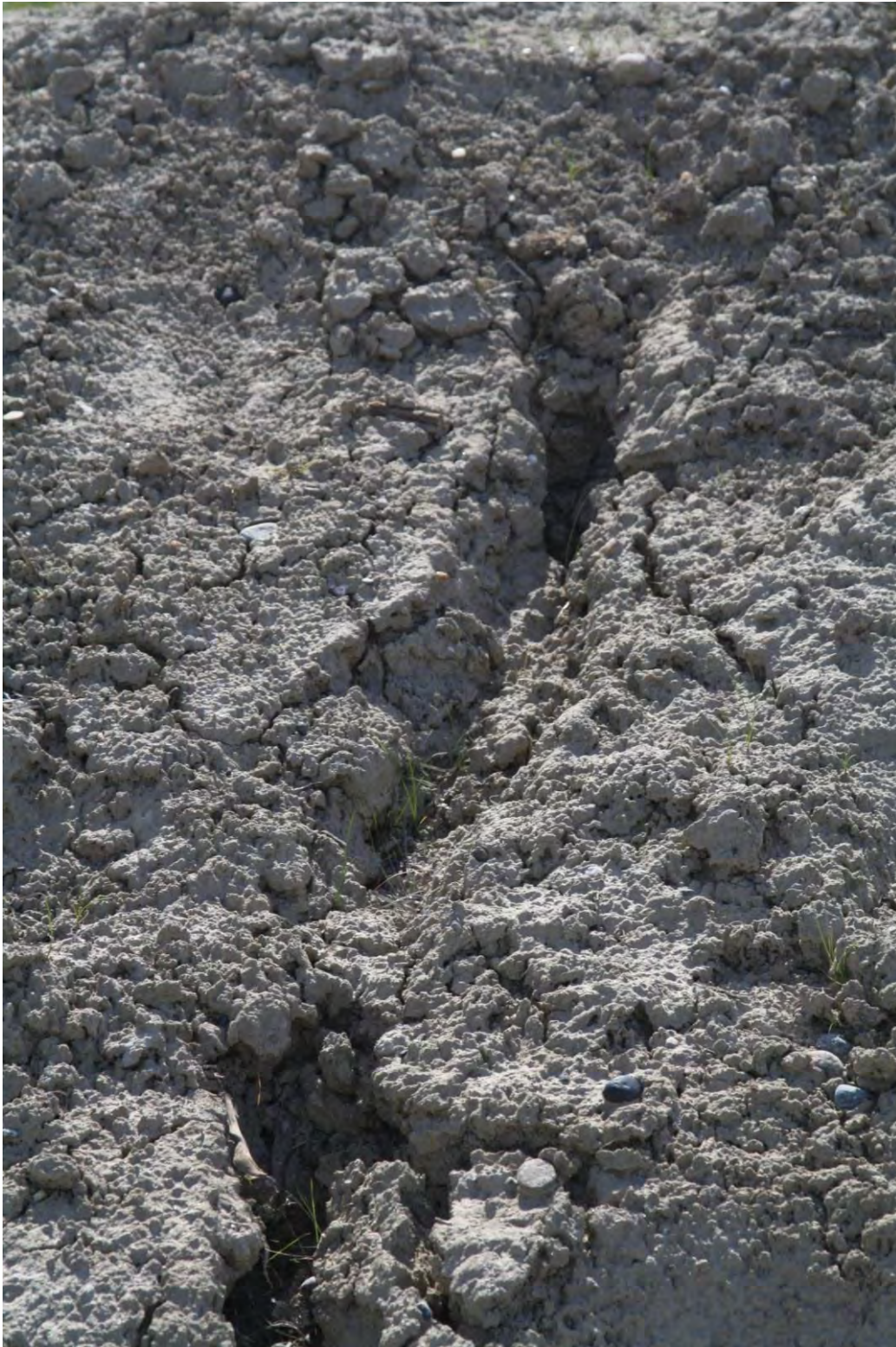
Fig. 4-7: Erosion on the backside of the constructed test site. An illustration of erosion when soil was not covered by plants or addition of dust-depressing materials (photo taken June 28, 2012)
