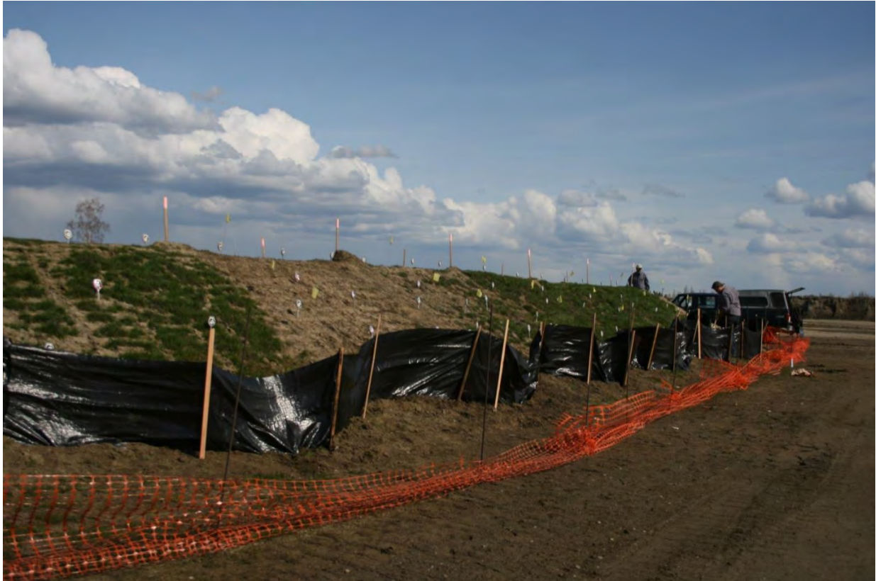
Fig. 3-17: Installed silt fence
