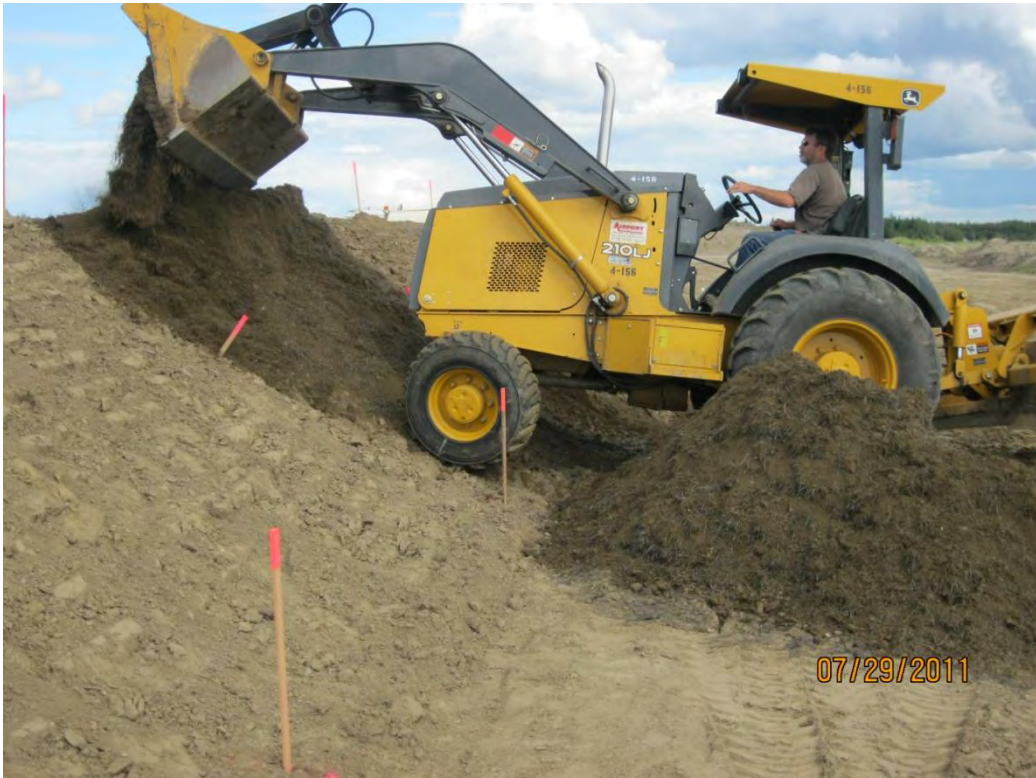
Fig. 3-12: Treated soil pushed onto side of slope
