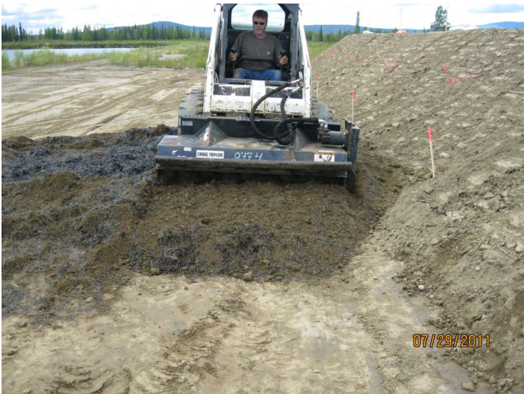
Fig. 3-11: Rototiller blending geofibers with stockpiled soils
