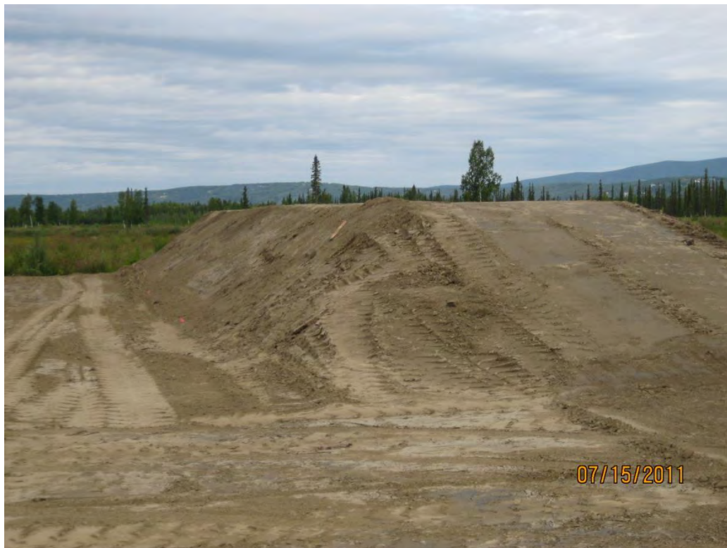
Fig. 3-6: Embankment prior to installation of test strips
