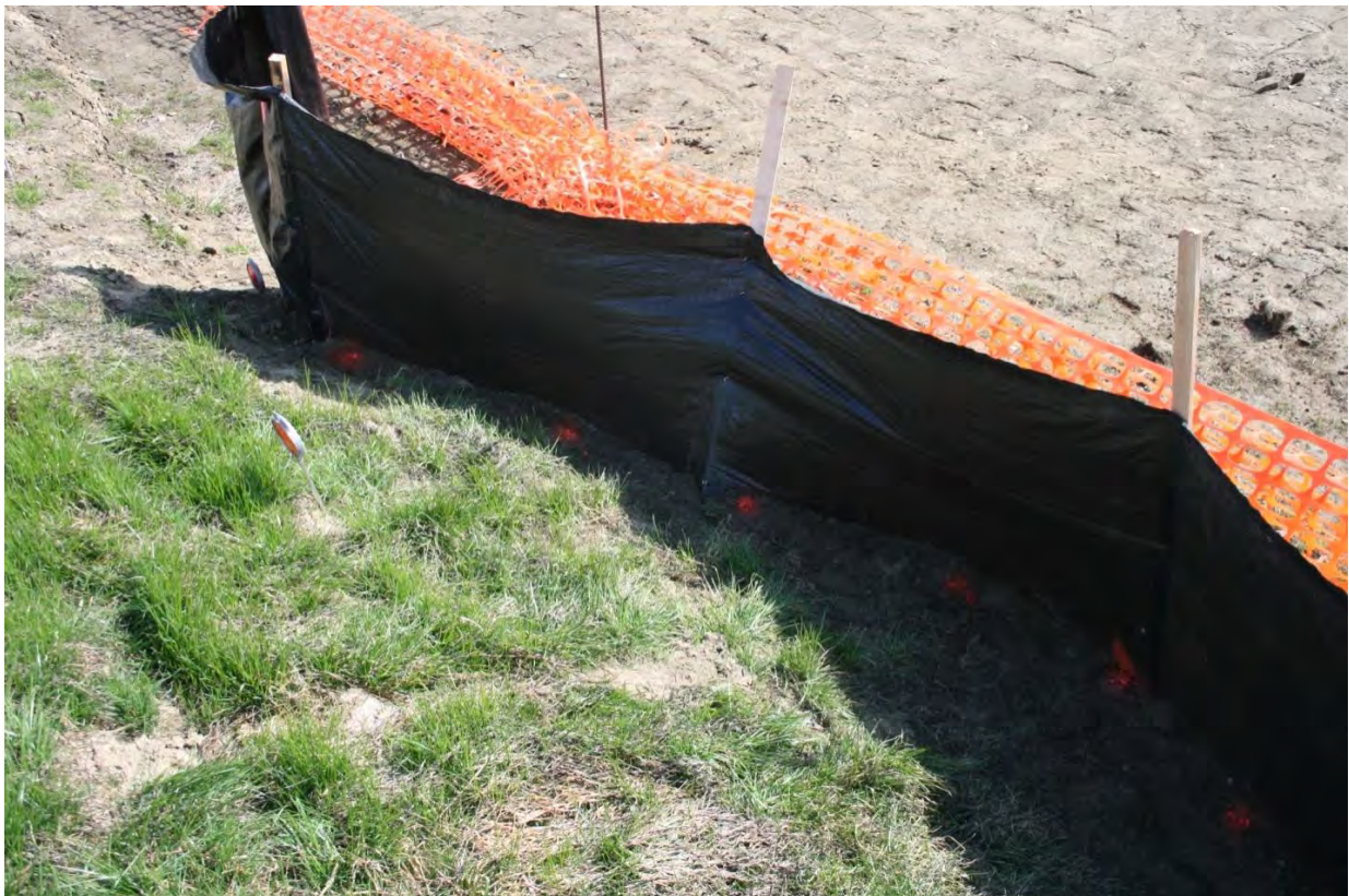
Fig. 3-18: Dots painted below base of silt fence allow for identification of runoff material from the slope
