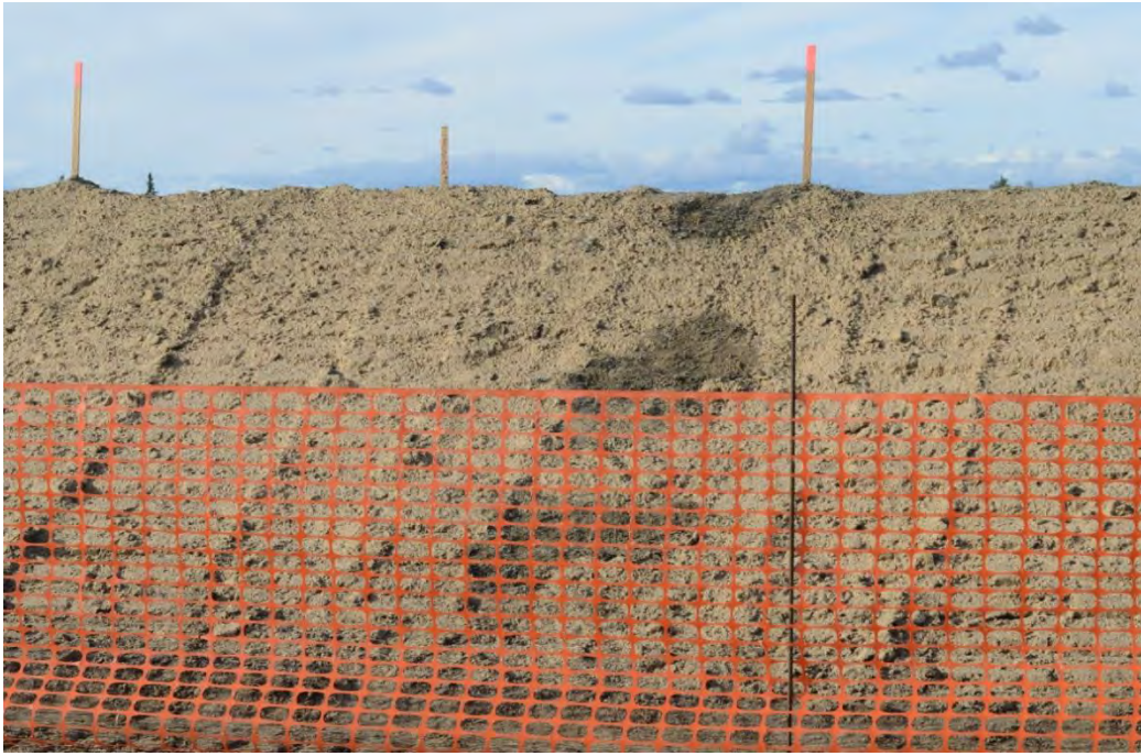
Fig. 3-14: Slope after hydroseeding
