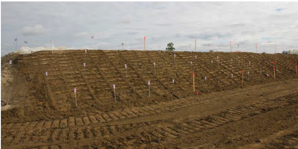
Fig. 3-7: Embankment compaction before treatment (south slope)
