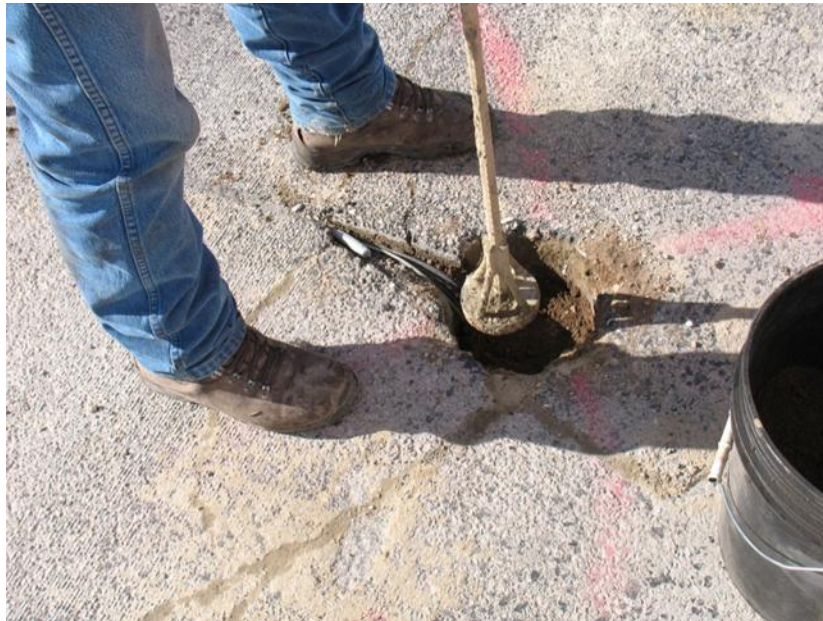
Figure 39. Photo. Kinniburgh Tamper Compacting Cold Mix to the Surface
