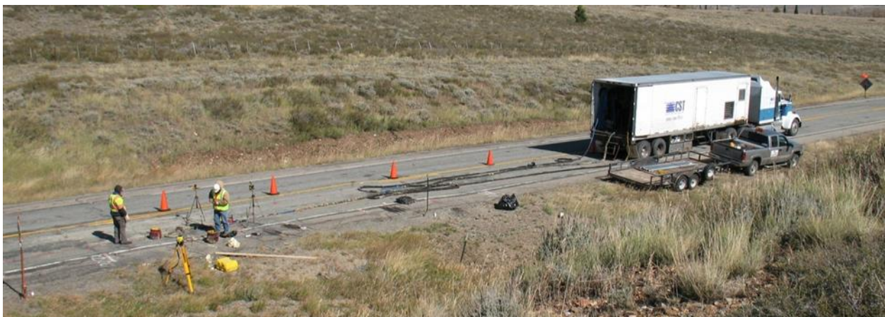
Figure 34. Photo. Site Layout showing the CST Urethane Truck, a Service Truck and Trailer, the Injection Hoses, the Leveling System and the Traffic Control
