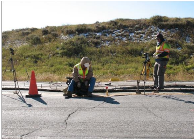
Figure 35. Photo. Injecting the Uretek at STA 2+10, the location of the dip. Also shown are some of the Injection Tubes.
