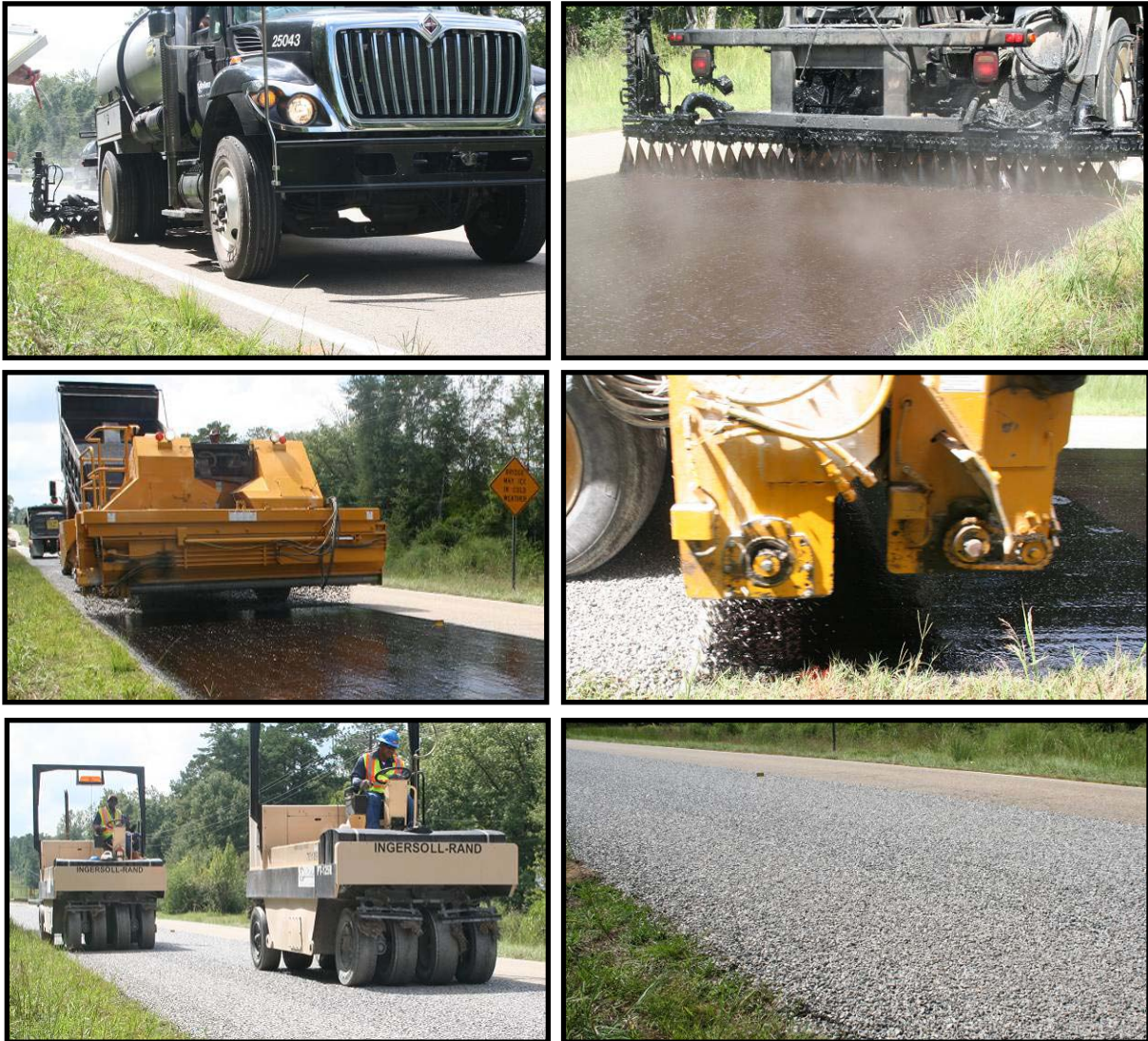
Figure 5.7. Hwy 44 Chip Seal Application (09/20/2011)
