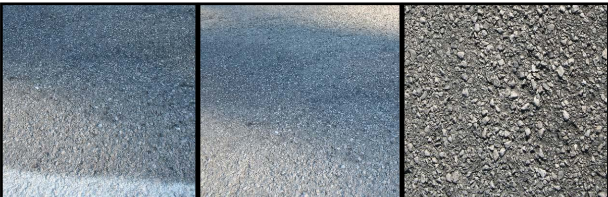
Figure 5.19. Hwy 366 Section 3 Intermediate Survey (06/27/2011)
