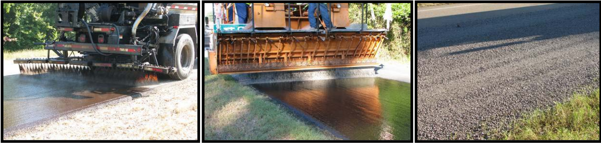
Figure 5.8. Hwy 366 Chip Seal Application (09/14/2010)
