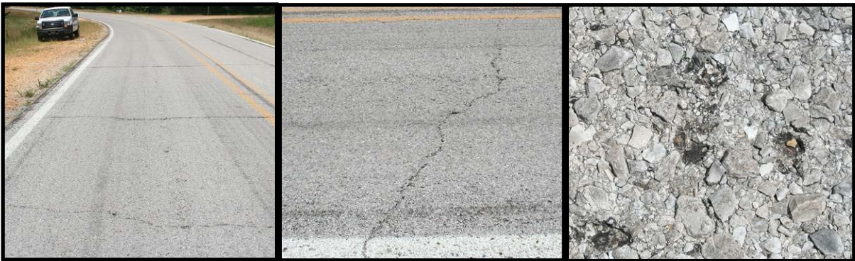
Figure 5.18. Hwy 366 Section 2 Intermediate Survey (06/27/2011)
